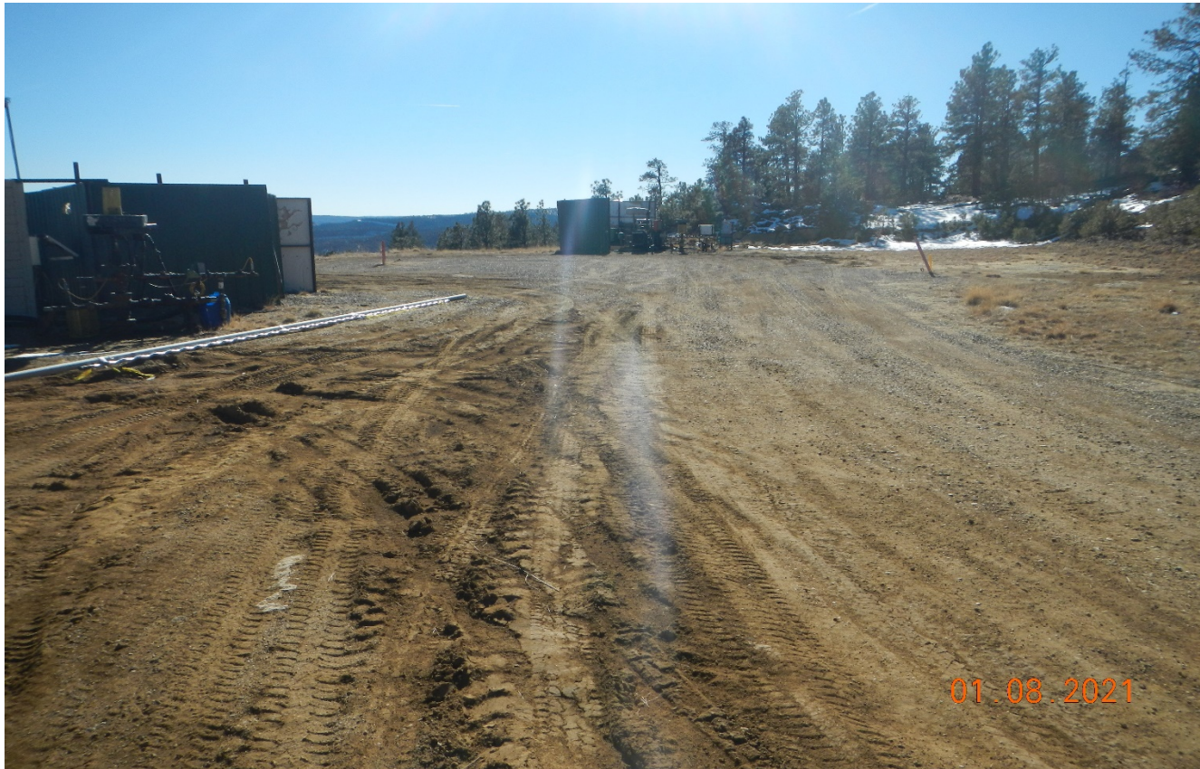
Photo 1. Facing southeast toward the location.
