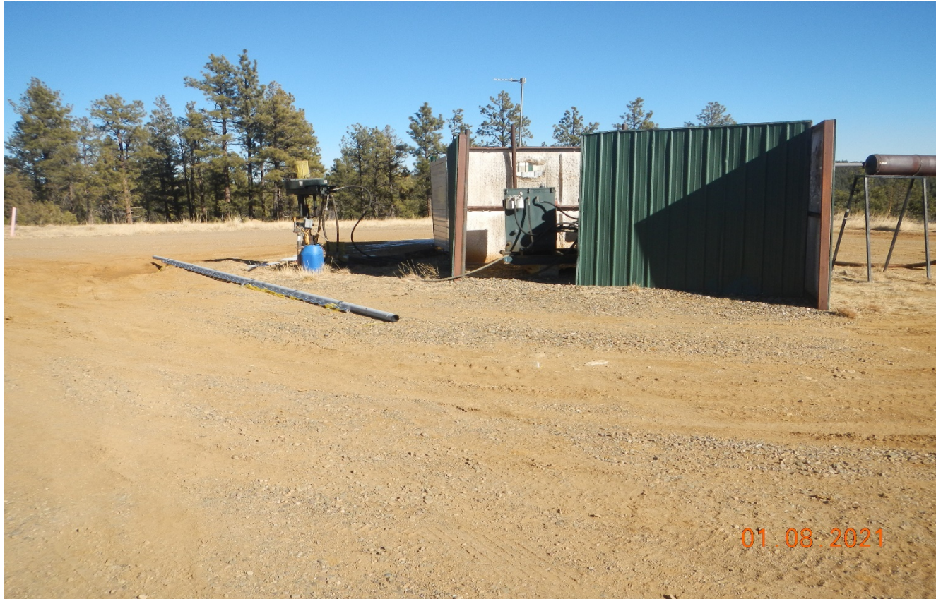
Photo 3. Facing toward the well. Unused pipe next to the well will need to be removed.
