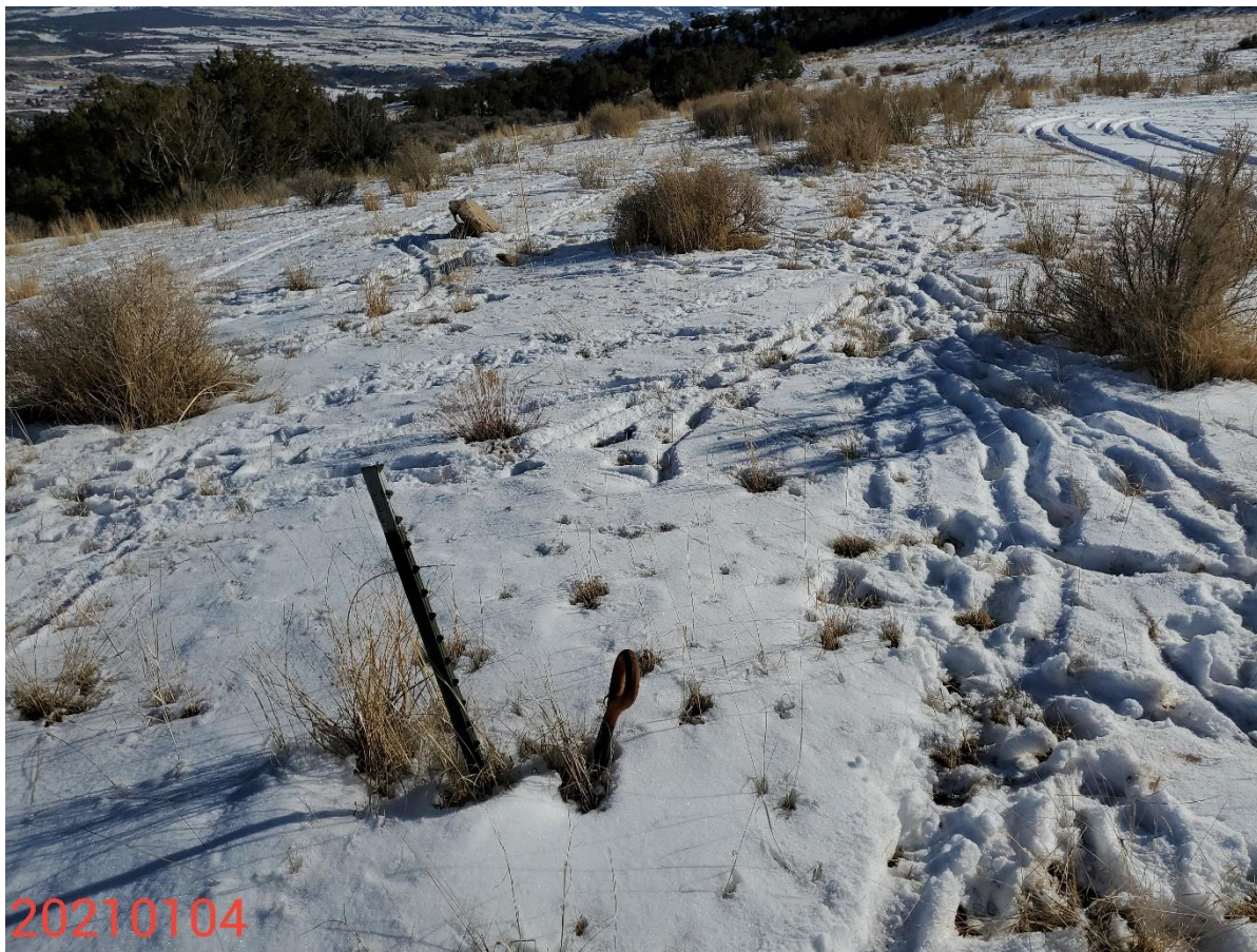
Photo 3: Photo taken from the east end of the Location, facing south. Photo shows example of marked anchors observed on the Location. Marker is not bright in color and at least 4 feet in height pursuant to Rule 1003.a
