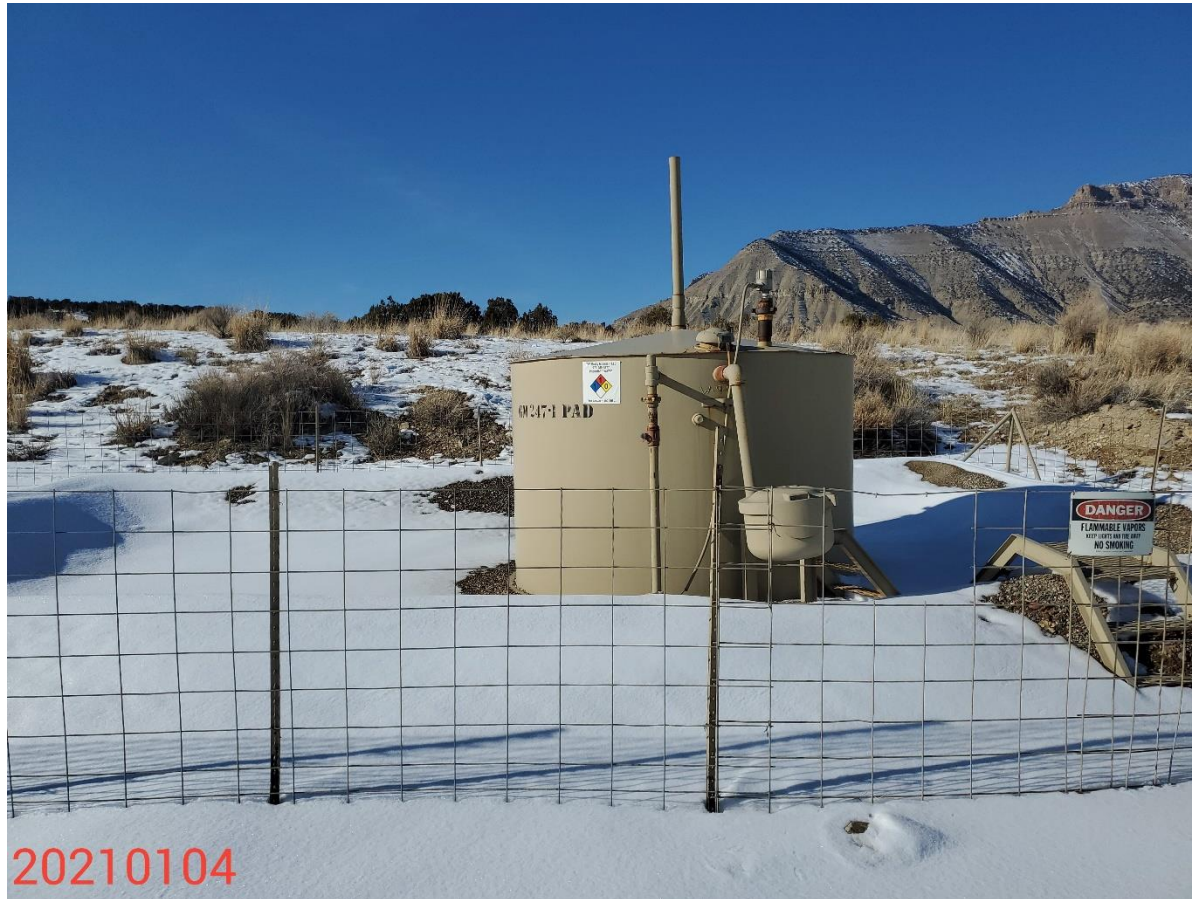
Photo 7: Photo taken from the north end of the 247-1 Location, facing north. Photo shows remote tank battery facility; 80 bbl Produced Water Tank
