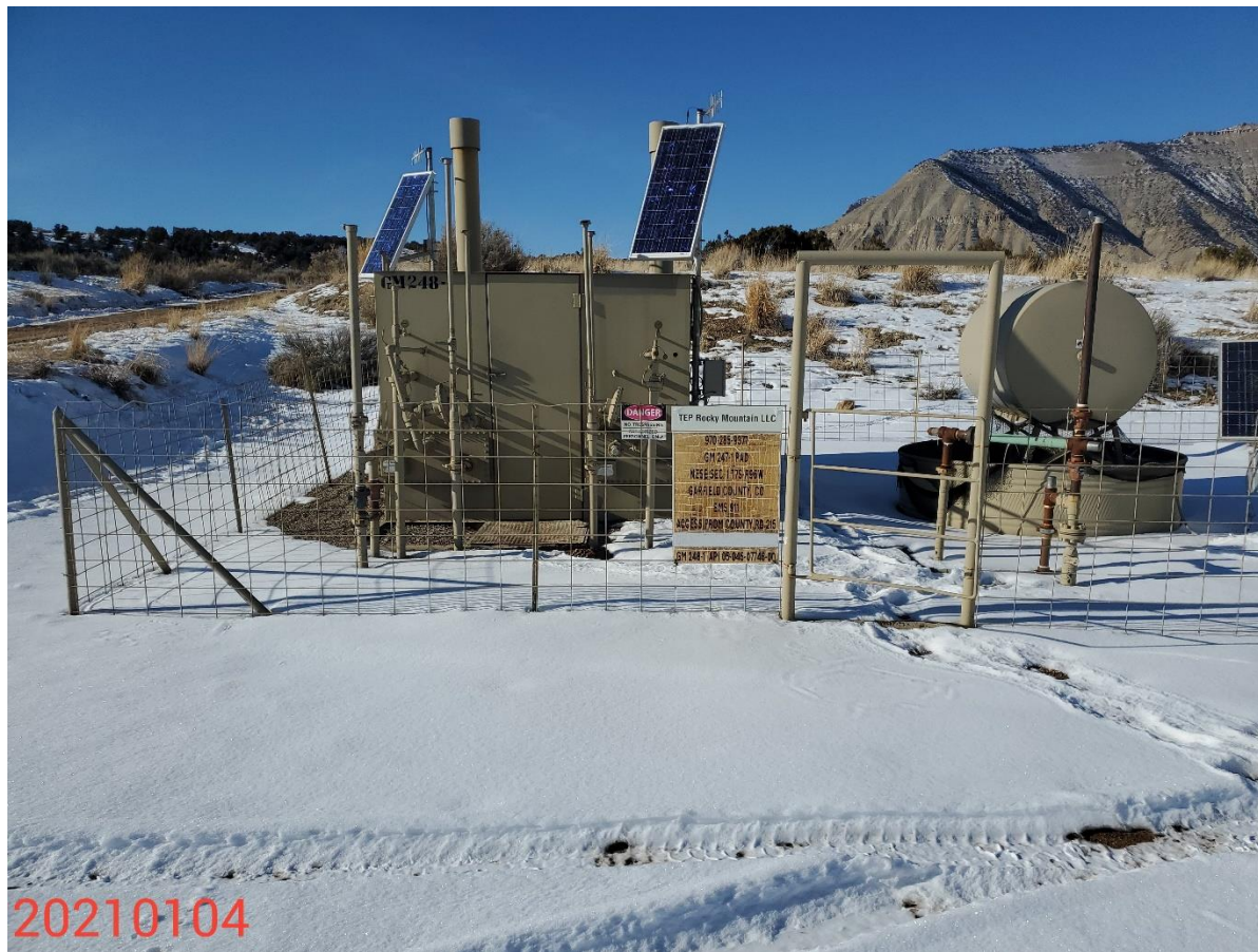
Photo 6: Photo taken from the north end of the 247-1 Location, facing north. Photo shows remote tank battery facility; Separator equipment and Methanol tank.
