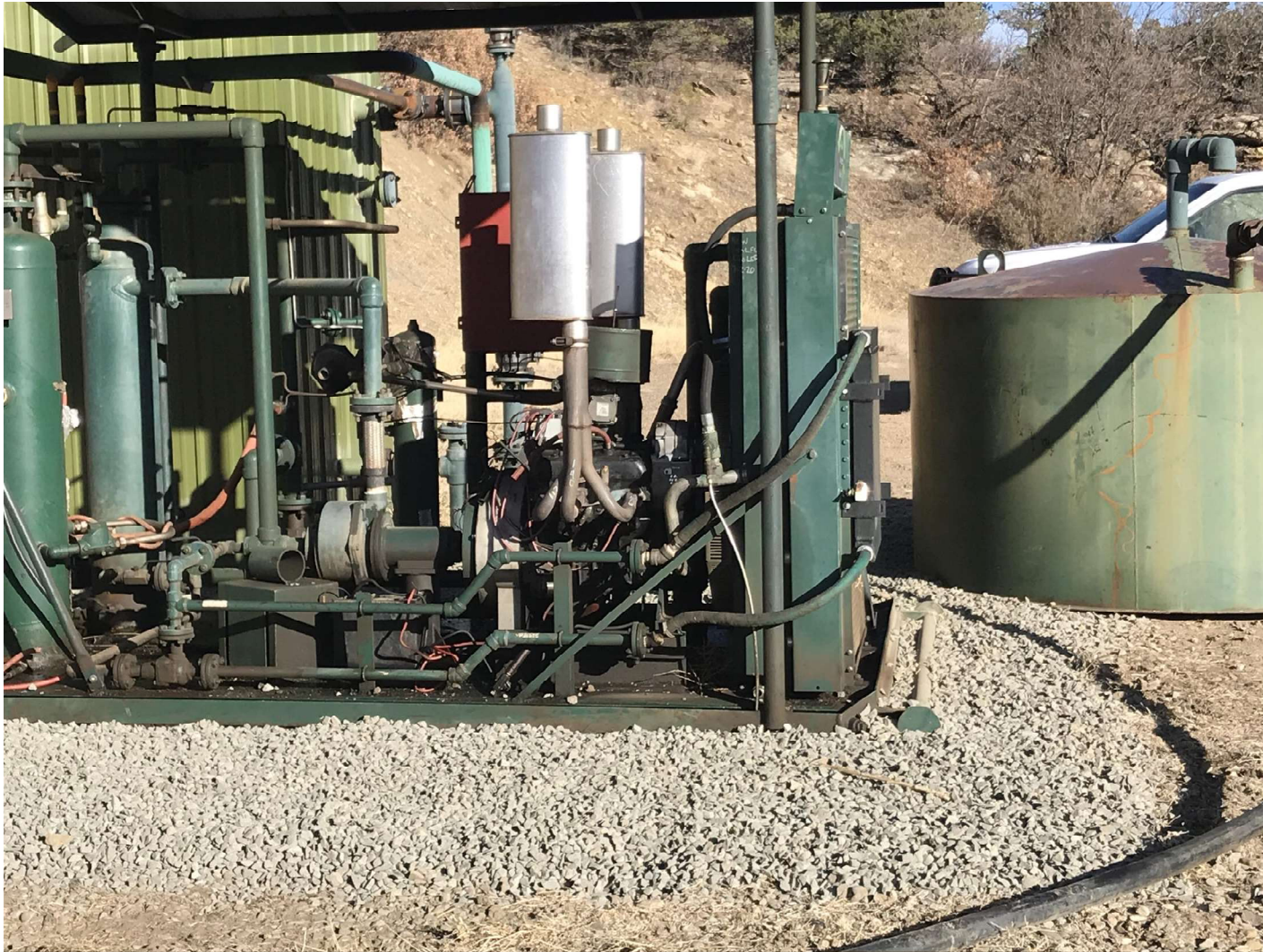
PHOTO 3: THE FLUID ACCUMULATION WAS REMOVED FROM THE CONTAINMENT OF THE LIQUID RING COMPRESSOR AND THE SKID WAS CLEANED UP.
