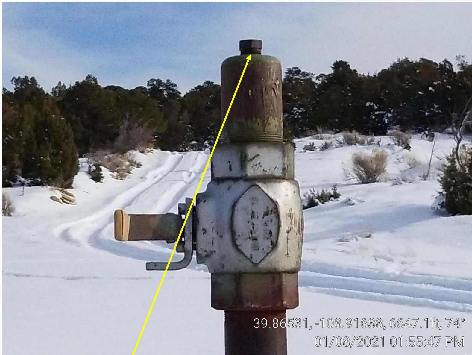
Photo 3. Gas leak at well.
