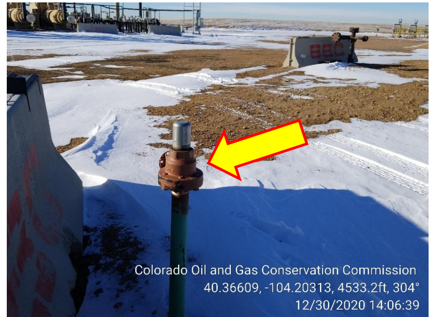
Photo 8 – Unmarked Riser at Soundwall
