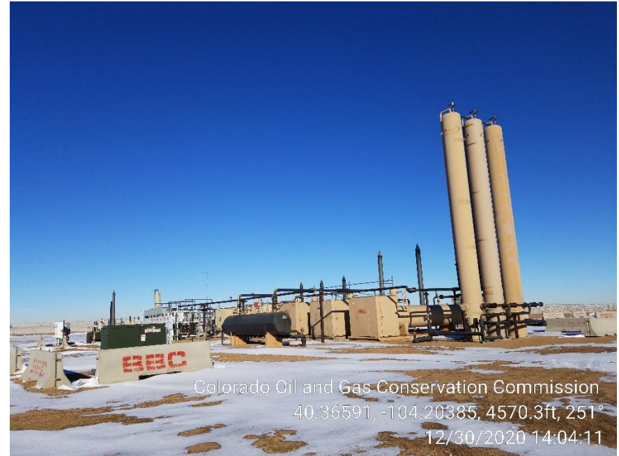
Photo 4 – Separators and VRT
