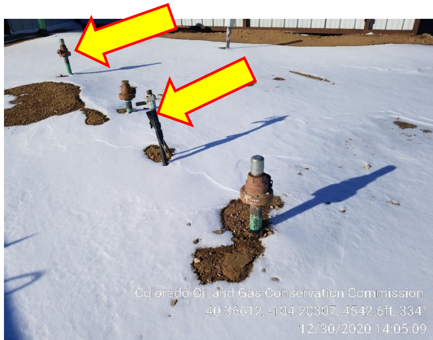
Photo 5 – Unmarked Risers at Soundwall
