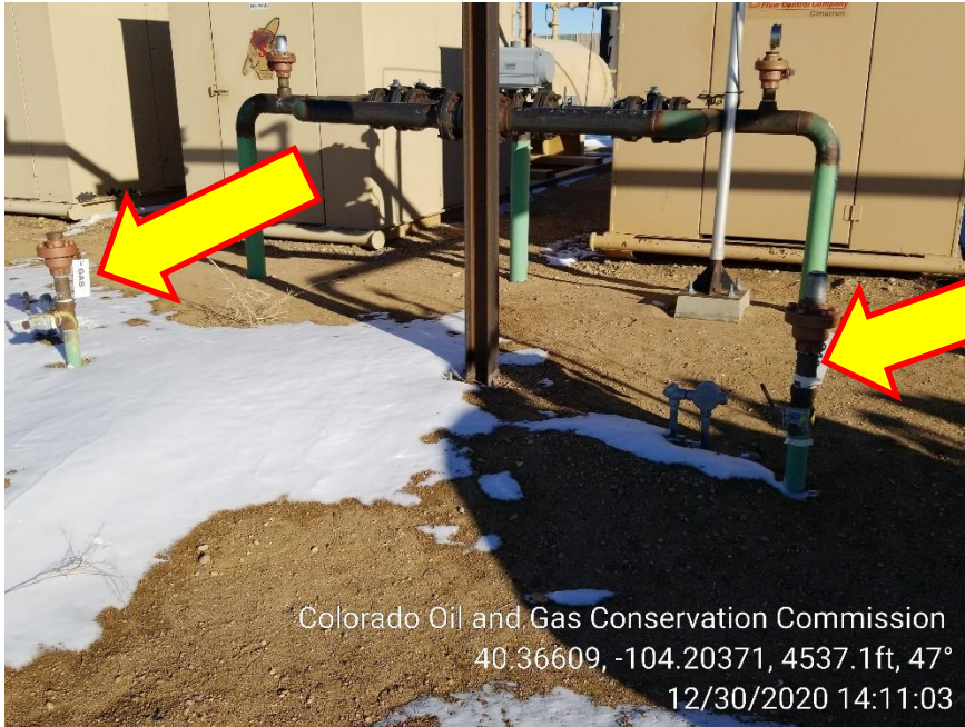
Photo 9 – Risers at VRUs have been marked
