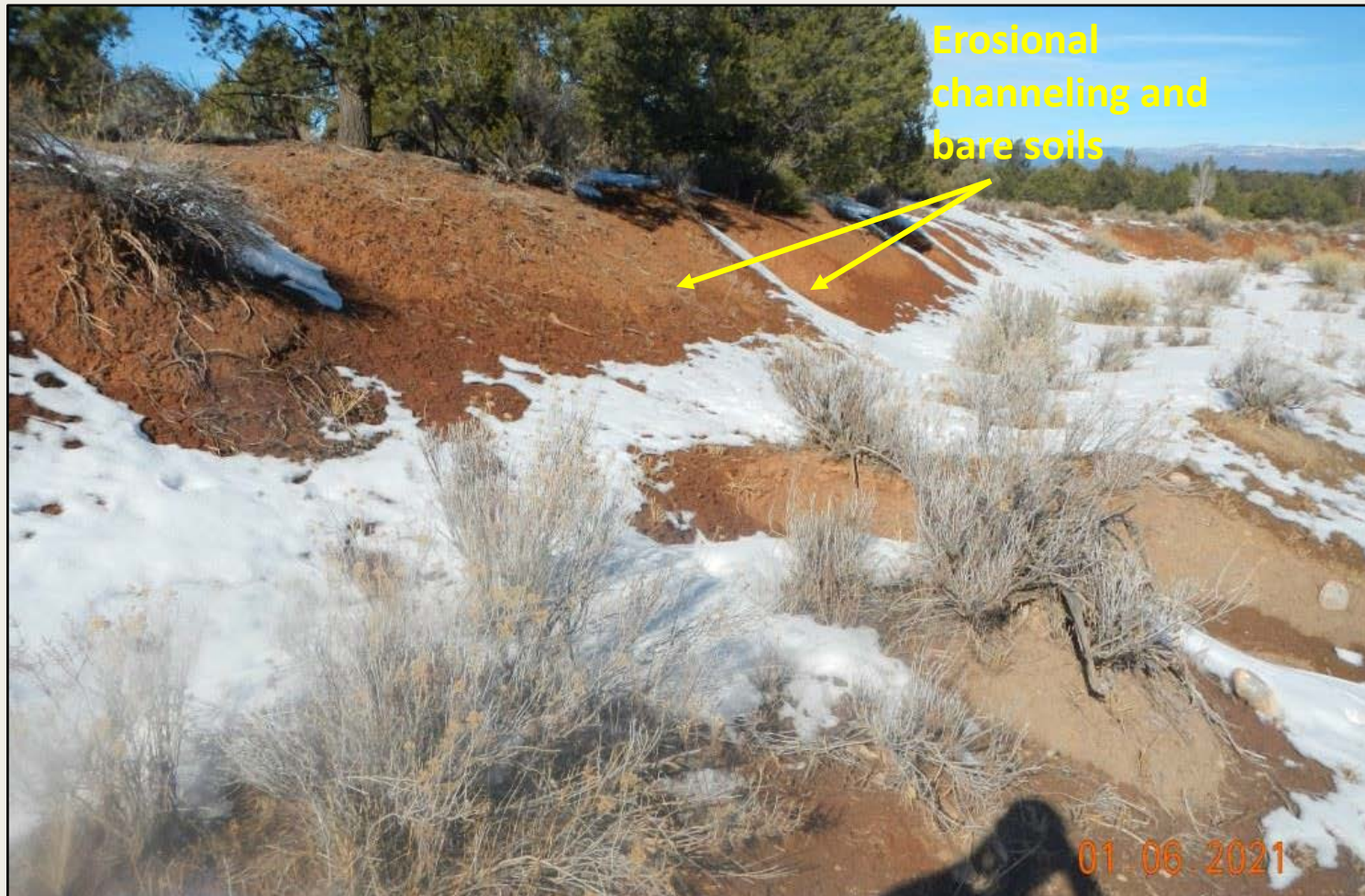
Photo 2. View of the western cut slope facing northward. Evidence of erosional channeling and bare soils observed. Cut slope was not recontoured.
