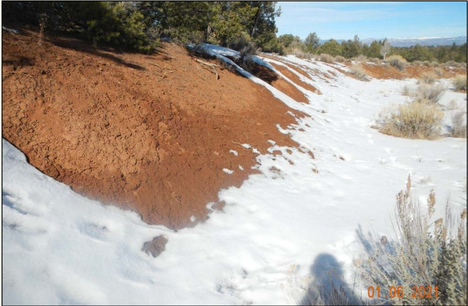
Photo 3. Another view of bare soils and steep cut-slopes lacking recontouring.
