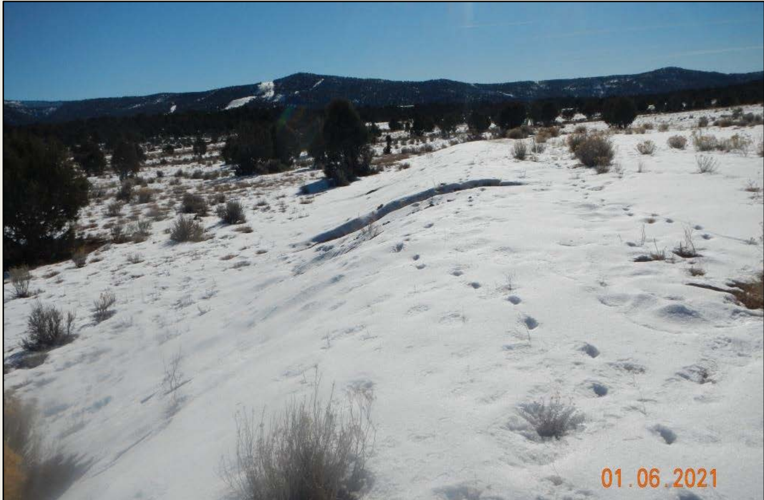
Photo 2. View of the eastern fill slope from the northeastern corner facing southward. Location is largely snow covered. Erosional channels appear to be forming in the fill slope.
