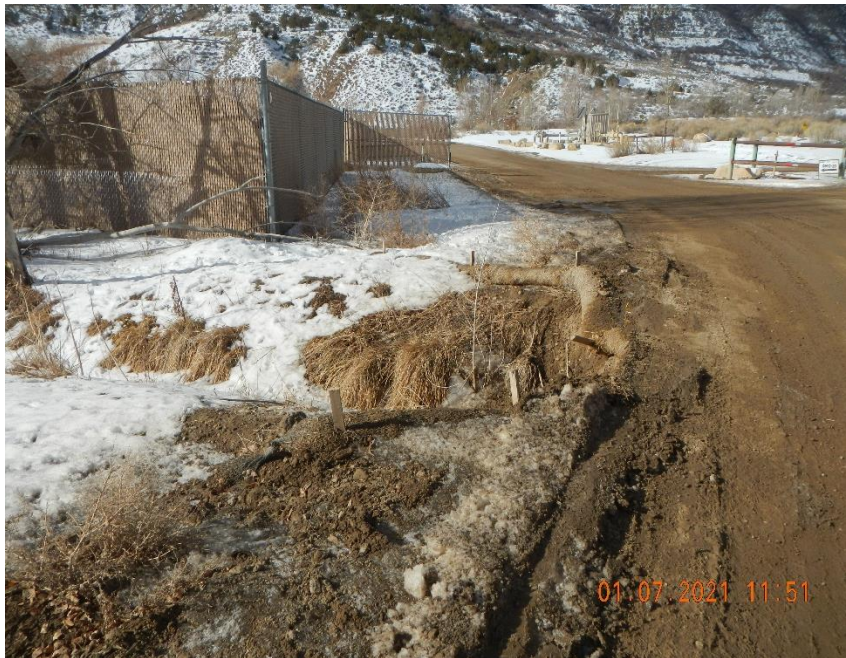
Culvert at intersection before the bottom guard shack has waddle that's damaged and sediment in ditch/culvert outlet
