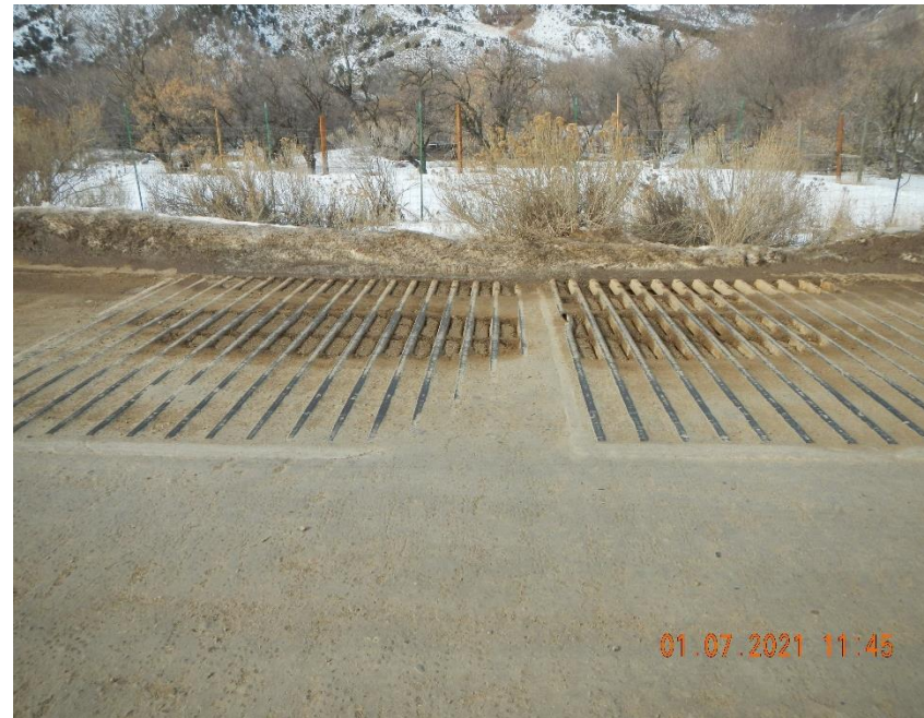
Sediment build up inside of tracking cattle guard style tracking pad.
