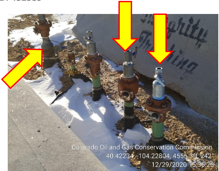
Photo 6 – Unmarked Risers
