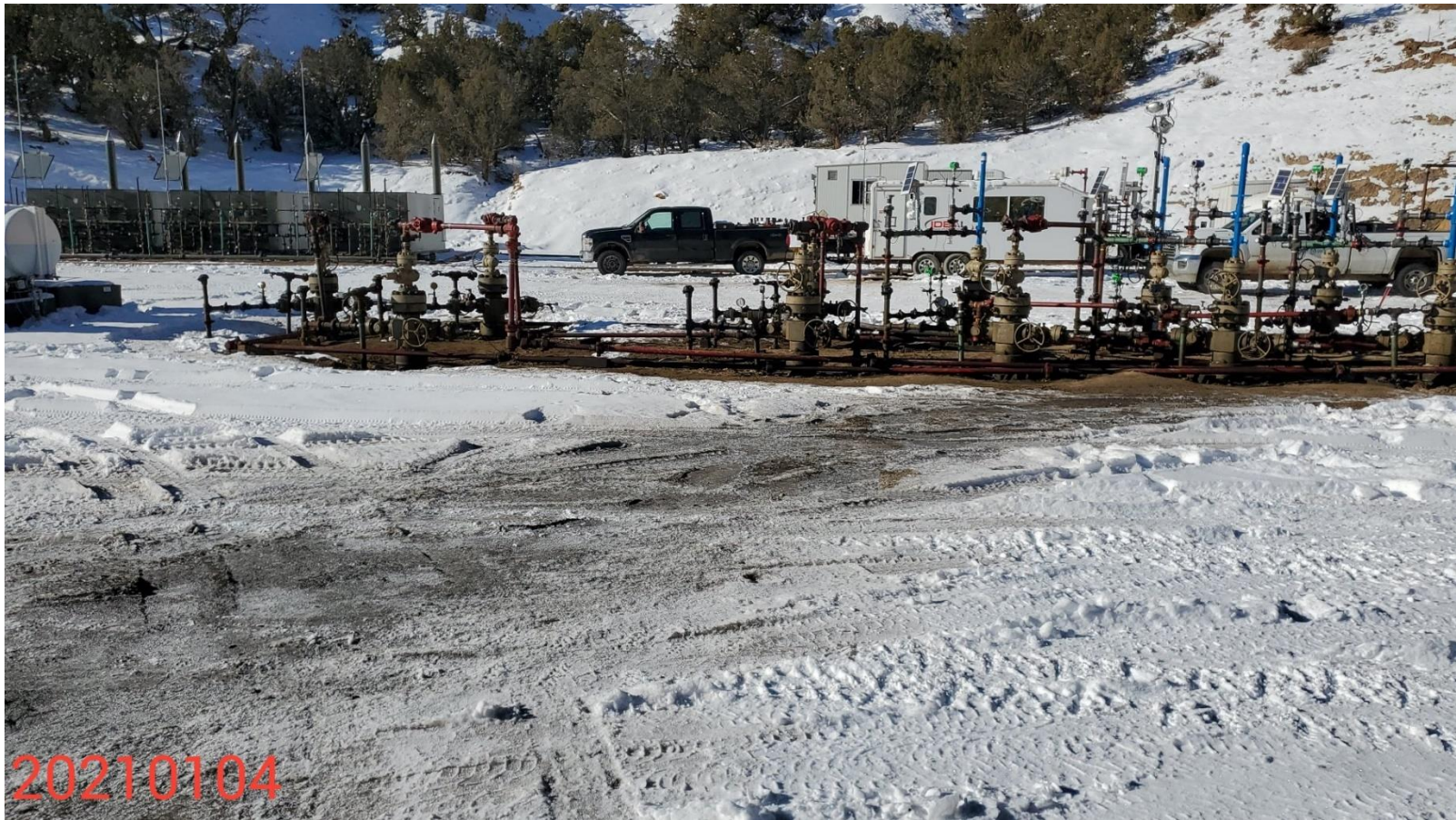
Photo 8: Photo taken from the Location, facing west. Photo shows wells; All permitted wells on the Location have been drilled; wells on Location missing signage. Signage due within 60 days of completion per Rule 210.b.(2)
