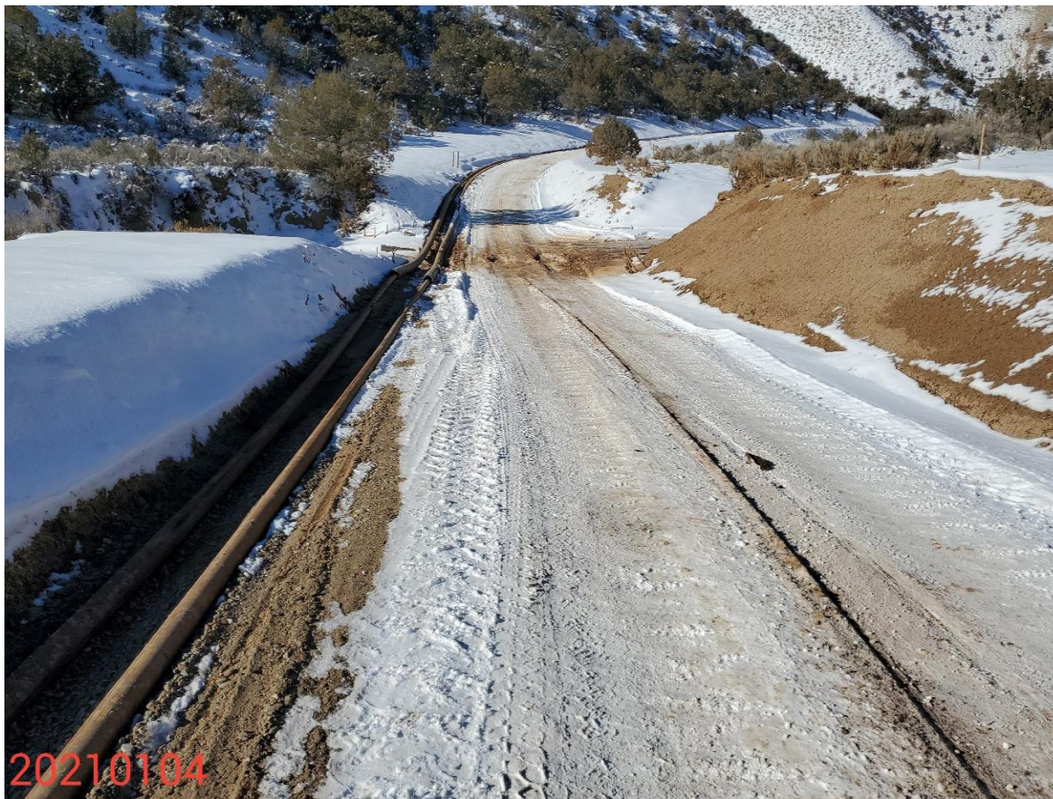
Photo 13: Photo taken from the access road at the stream crossing, facing west. Photo shows proper BMPs per good engineering practices remain missing, or insufficient to stabilize access road at stream crossing
