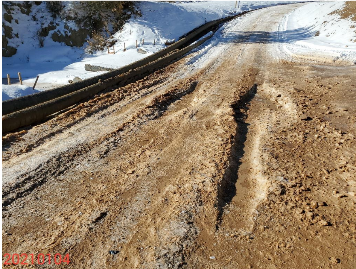
Photo 16: Photo taken from the access road at the stream crossing, facing west. Photo shows proper BMPs per good engineering practices remain missing to protect the waterway and stabilize access road at stream crossing
