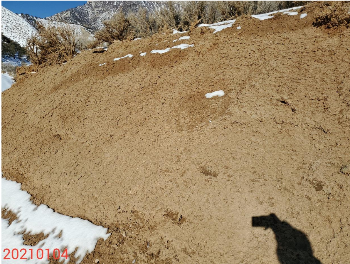
Photo 14: Continued from photo 13. Photo shows Operator installed hydromulch on slopes along areas cut during construction of the access road.
