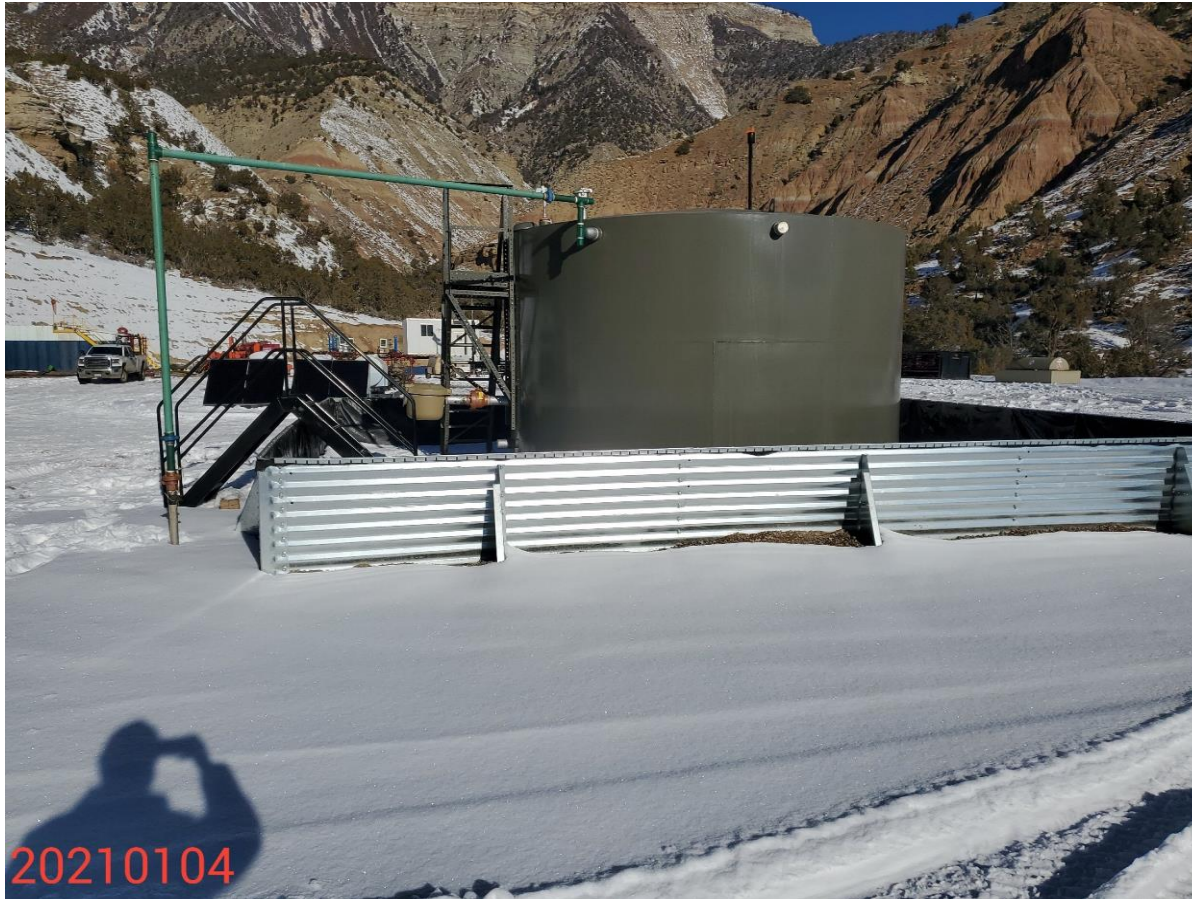
Photo 7: Photo taken from the south end of the Location, facing north. Photo shows tank on Location missing signage and labeling. Signage due within 60 days of installation per Rule 210.b.(2). Labeling required on tanks per 210.d.(1).
