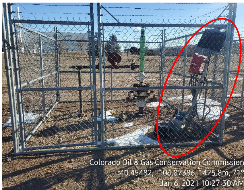
Photo 1: Wellhead; No sign, disconnected automation
