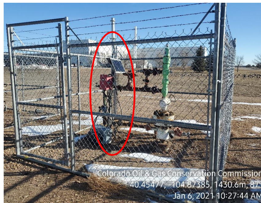
Photo 2: Wellhead; No sign, disconnected automation
