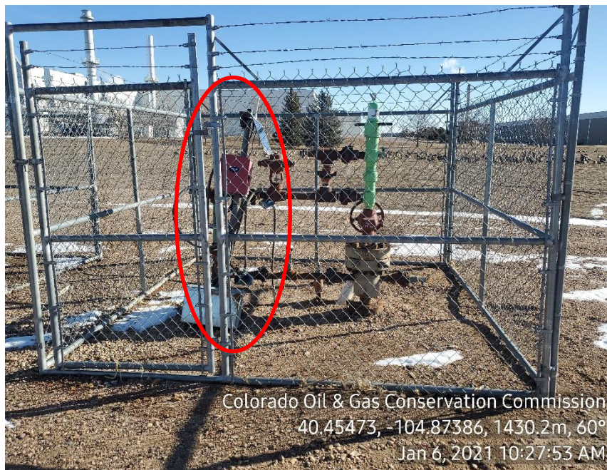
Photo 3: Wellhead; No Sign, disconnected automation
