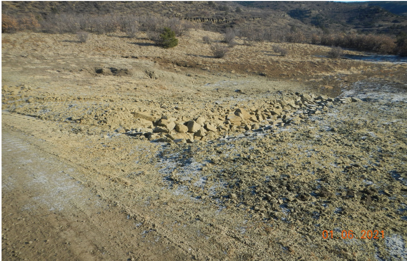
Photo 4. The erosion at the culvert outlet was repaired and outlet protection installed.
