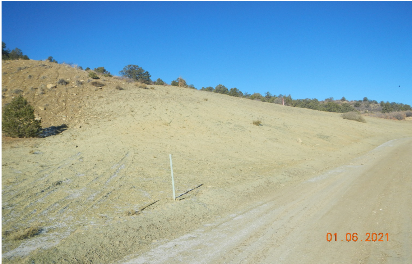
Photo 2. Facing northwest toward the location. The fill slope of the location was seeded and hydromulched.
