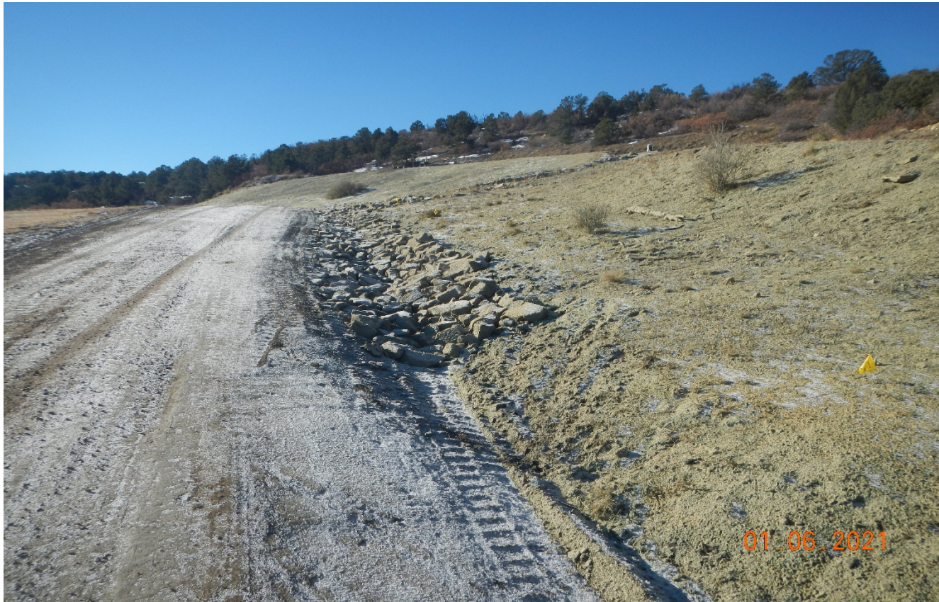
Photo 3. Facing southwest along the main road. Erosion along the road has been repaired.
