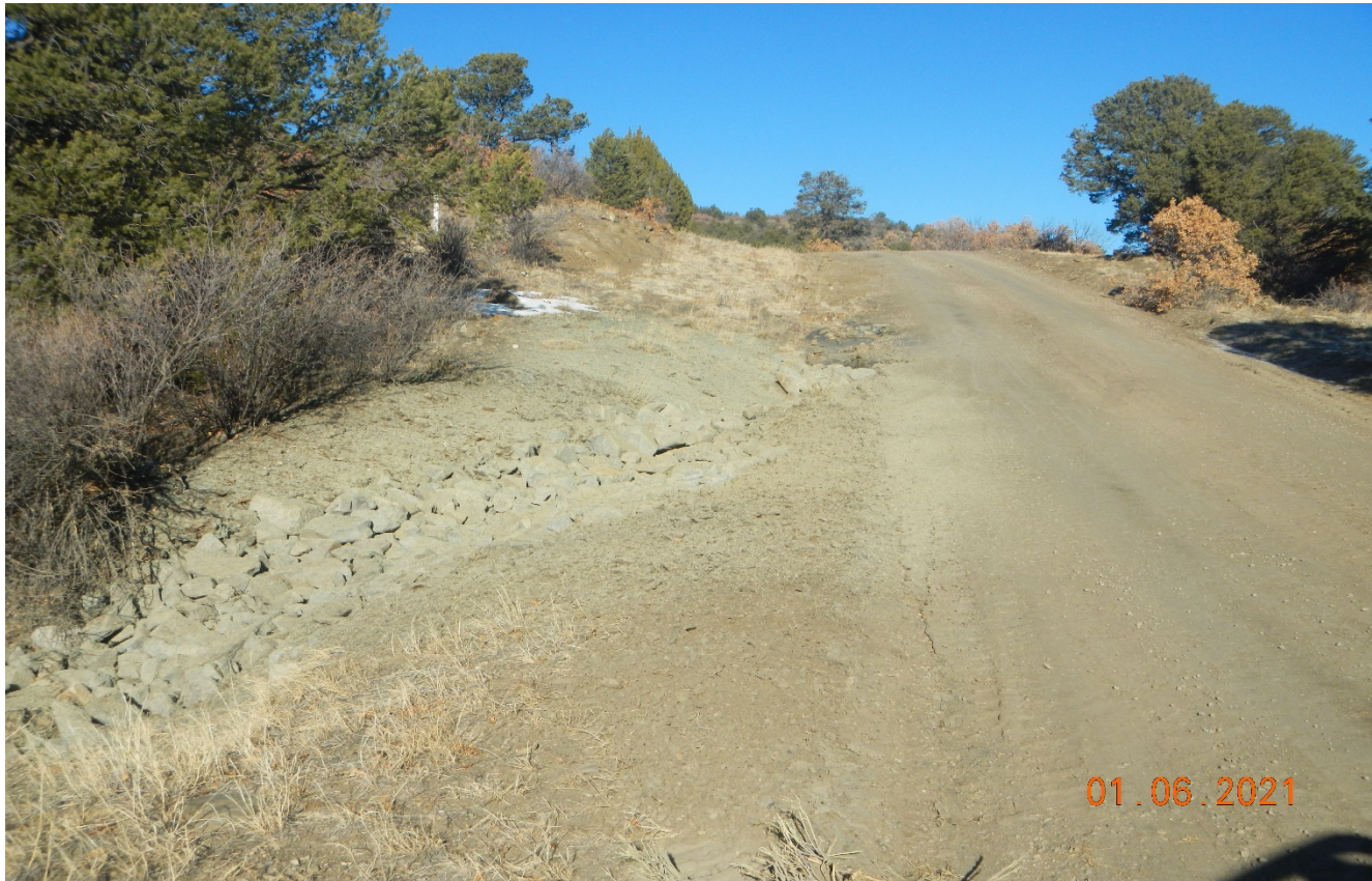
Photo 1. Erosion along the main road has been repaired.
