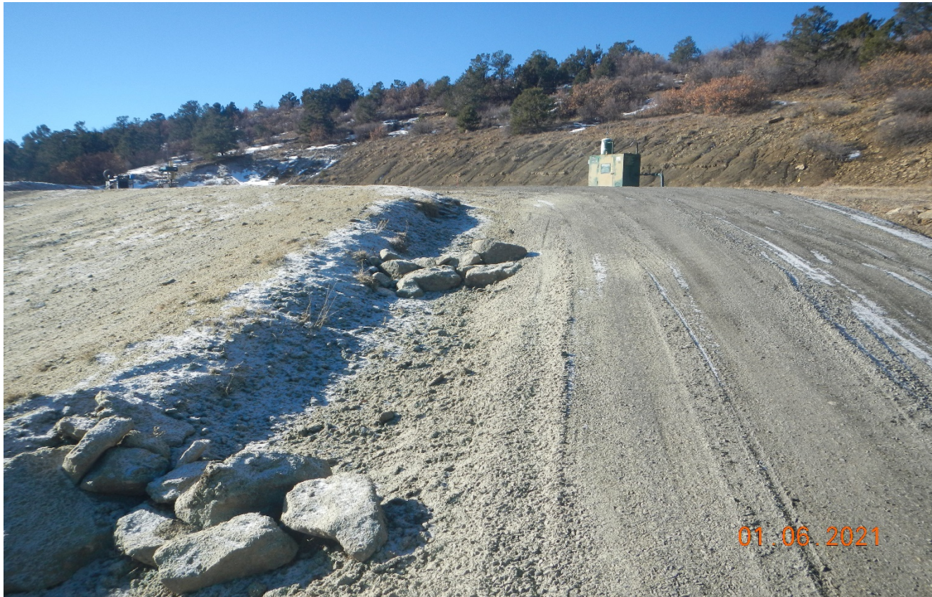
Photo 5. Facing southwest toward the location. Erosion has been repaired and BMP's installed.
