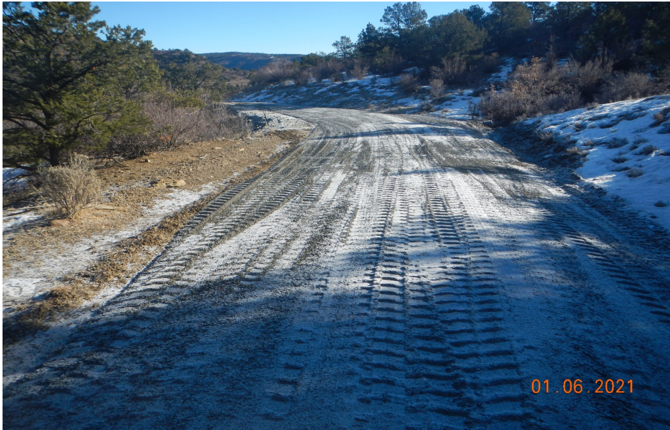
Photo 1. Facing east. Erosion along the access road has been repaired and culverts maintained.
