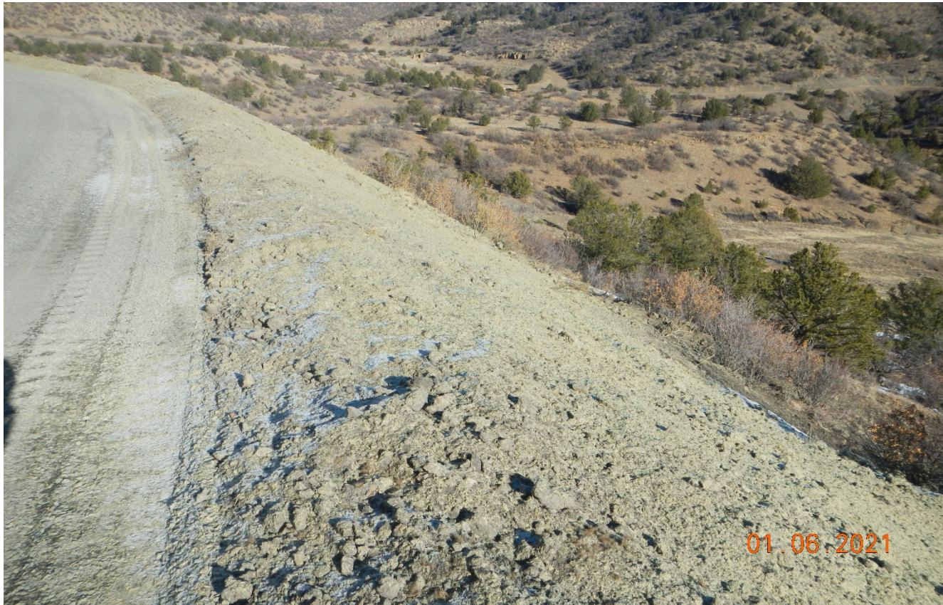
Photo 3. The erosion along the fill slope of the road has been repaired and stabilized.
