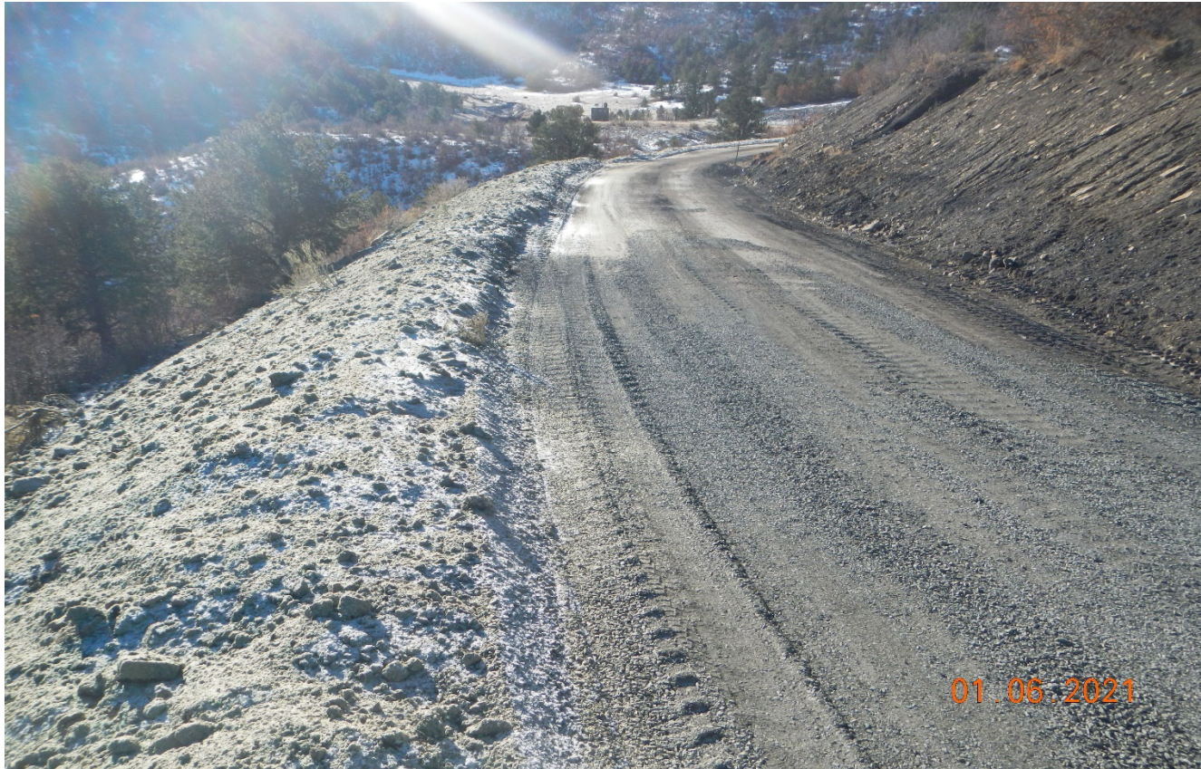
Photo 4. Facing south along the access road. Drainage is directed toward the culvert.
