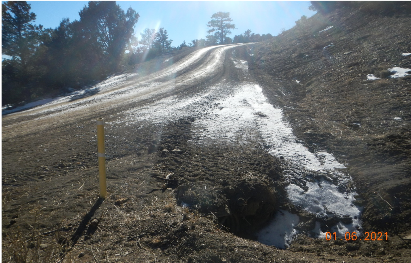
Photo 3. Facing south along the access road ascending the hillside. The culvert along the access road has been cleaned out and maintained.
