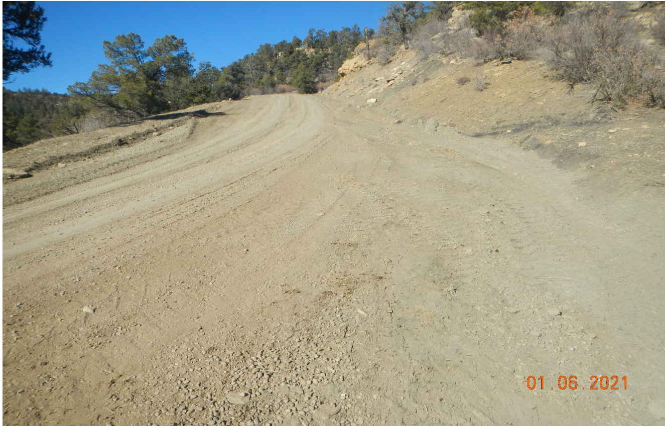
Photo 1. Facing northwest toward the access road. The erosion along the road has been repaired. Additional stabilization should be performed to prevent erosion.
