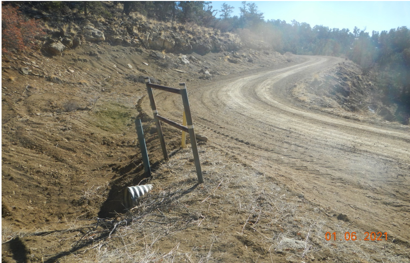
Photo 1. Facing southwest along the road. Culverts have been maintained and the road was graded.
