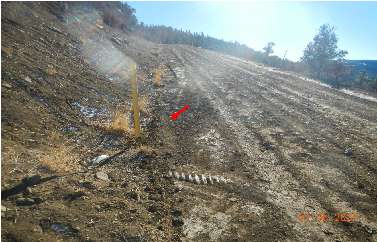
Photo 1. Facing south along the main road ascending the hill side. The road has been regraded. Red arrow points to dirt row which will prevent stormwater flow toward the culvert. Better diversion is needed.
