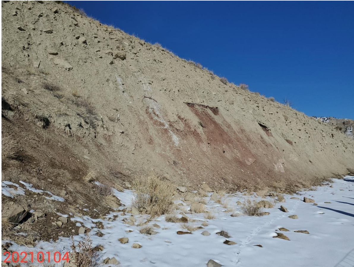
Photo 4: Photo taken from the north end of the Location, facing northeast. Photo shows cut slope. Erosion degradation and stability concerns observed. BMPs to stabilize/protect slopes missing or insufficient.
