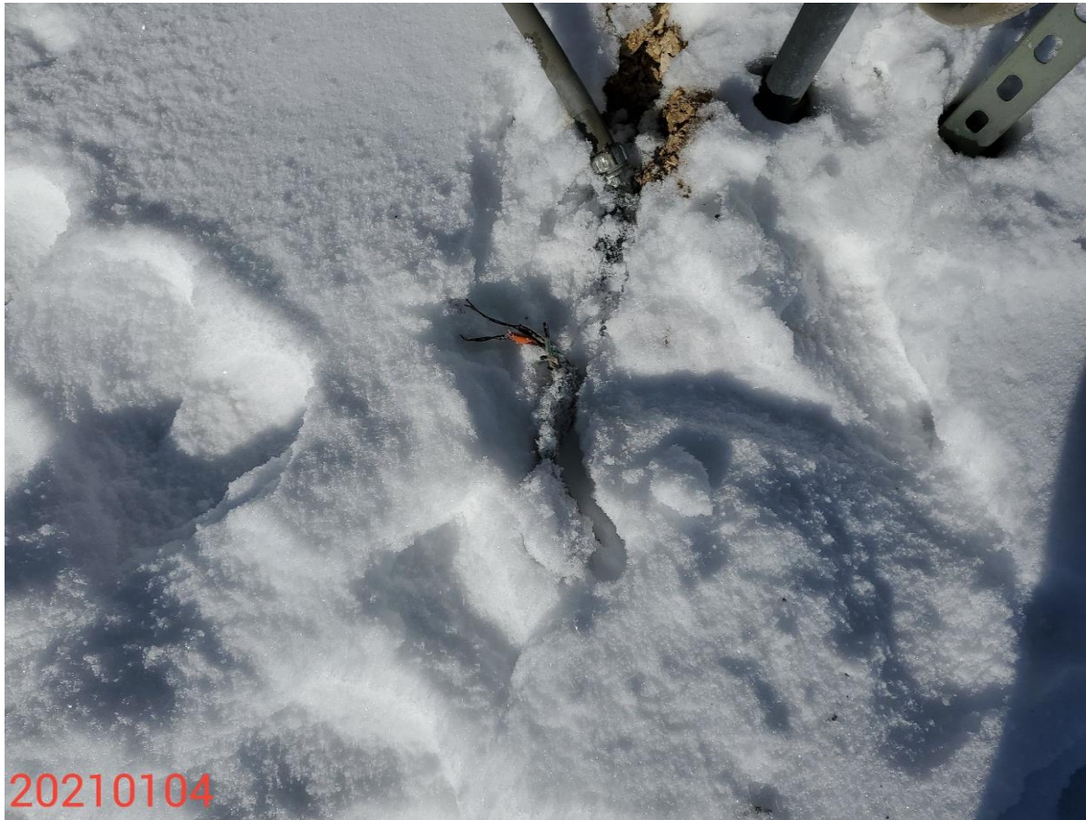
Photo 5: Continued from photo 4. Photo shows exposed electrical wiring.
