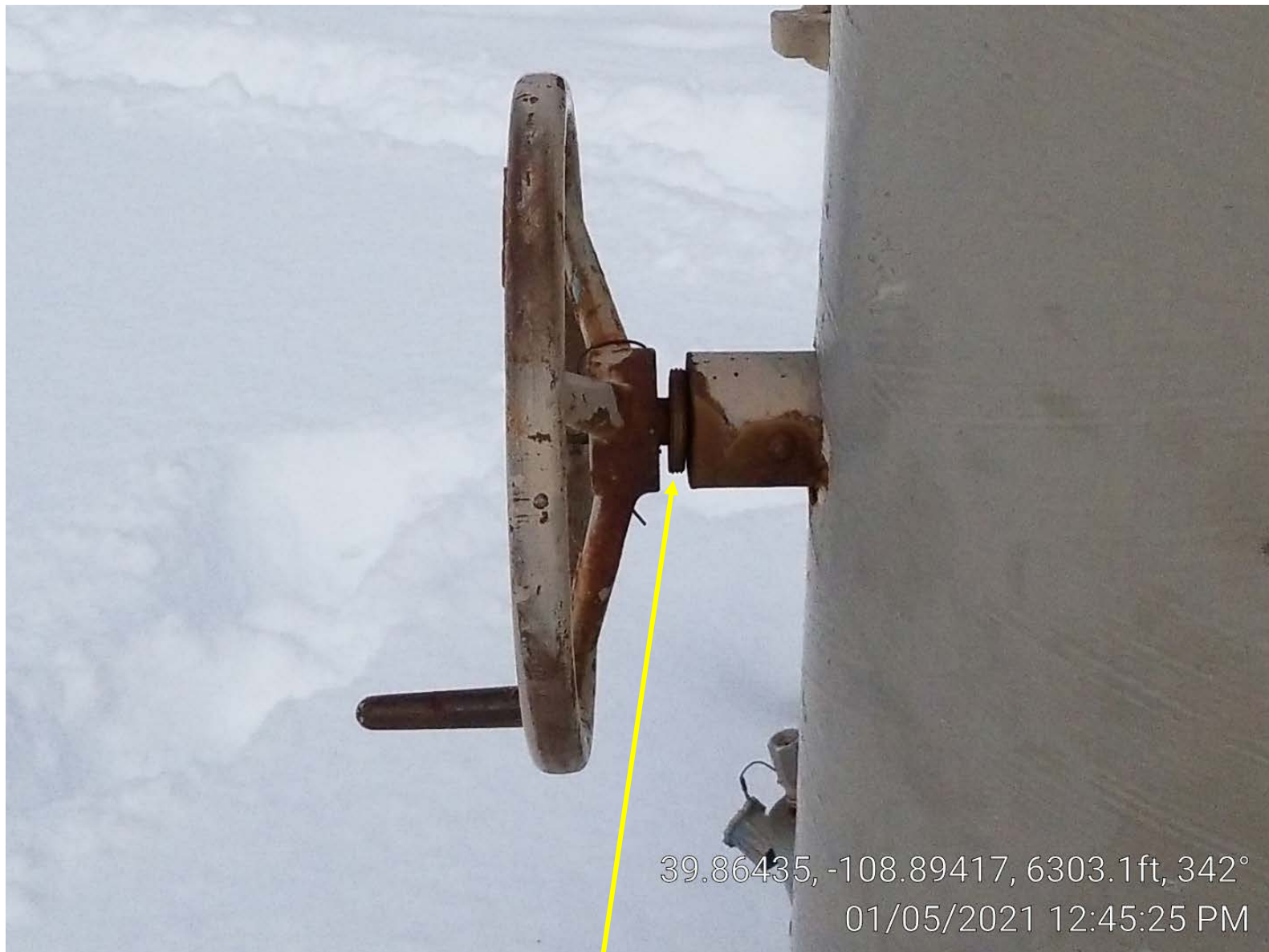
Photo 3. Wheel valve at well.
