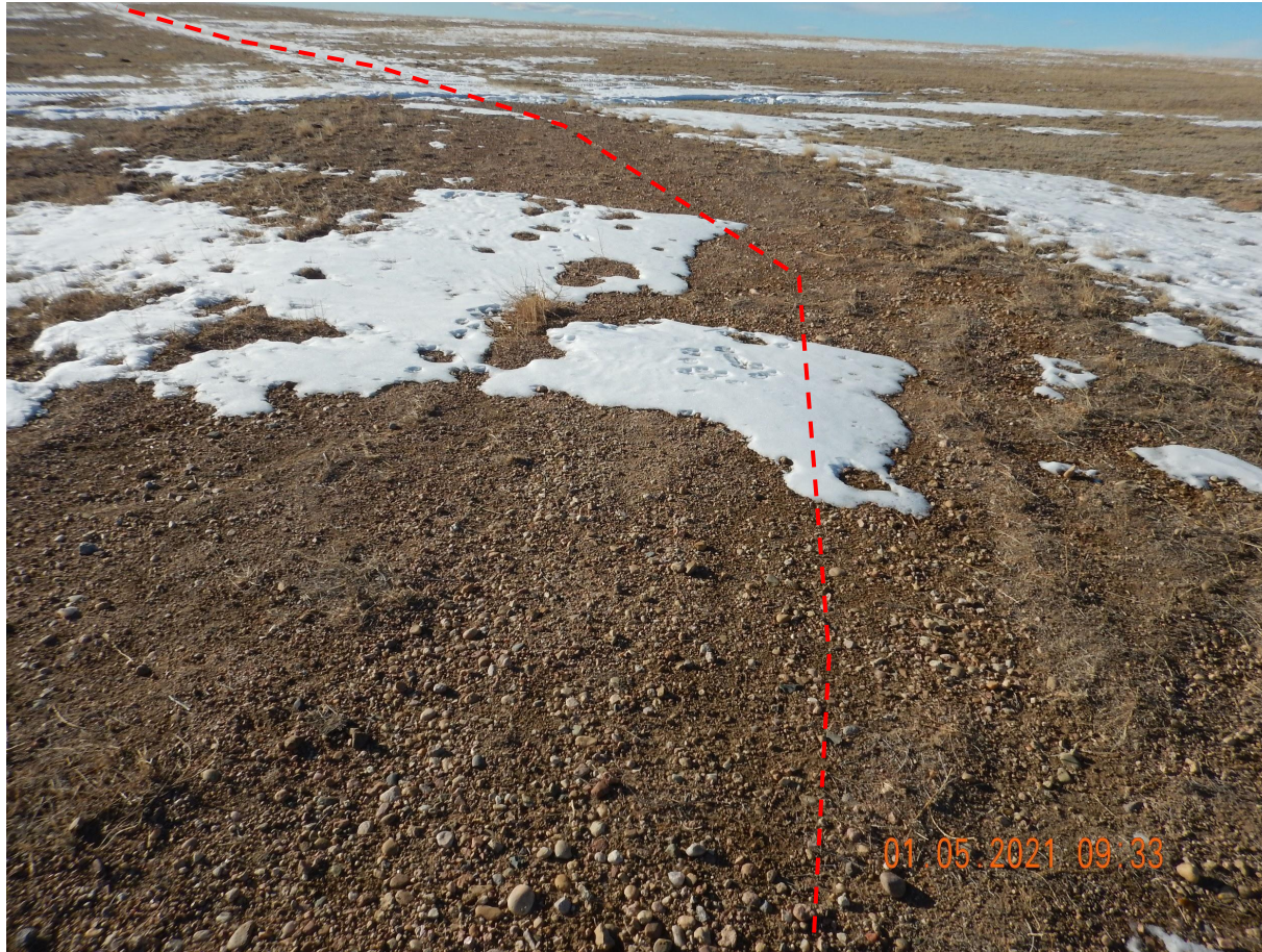
Photo 2. Photo taken from the northern access road, facing West. Photo illustrates the Operator has failed to remove gravel and perform final reclamation activities.
