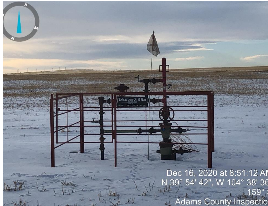
Photo #3 Well Head.
