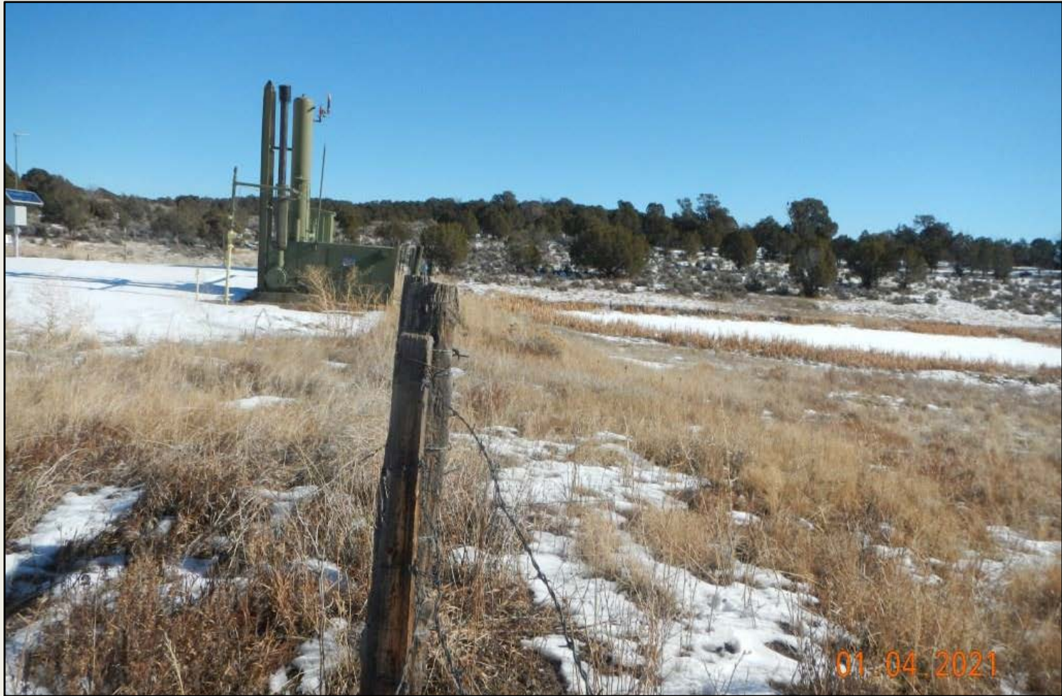
Photo 2. View of the southern fill slope from the southwestern corner facing eastward. Revegetation is progressing with grasses observed such as smooth brome, thickspike wheatgrass, and sideoats grama.
