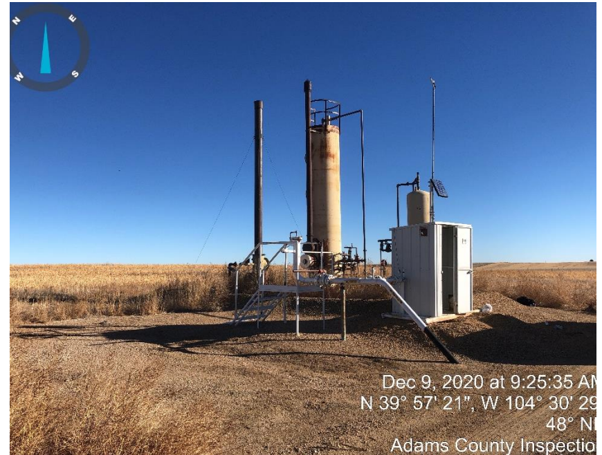
Photo #2 Separator, ECD & Meter run.
