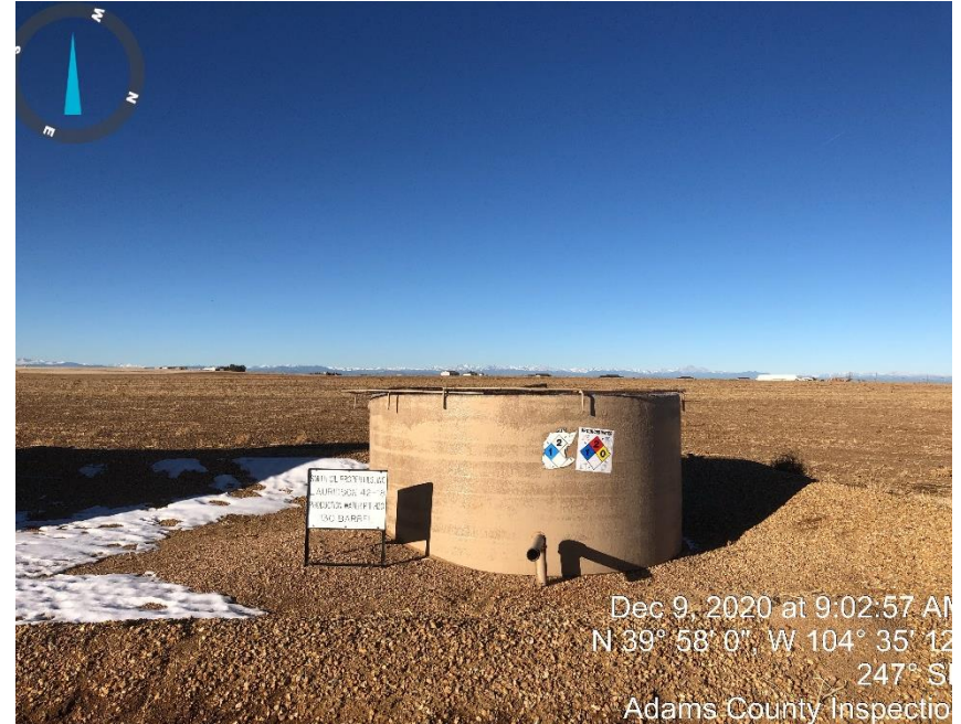
Photo #2 Produced Water Tank.
