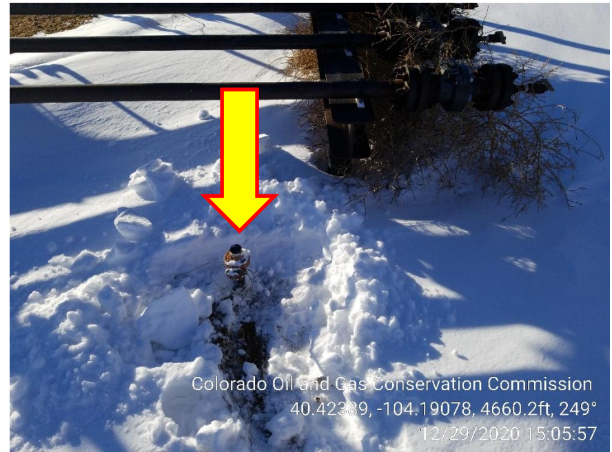
Photo 10 – Unmarked 1" Riser at North end of Rack
