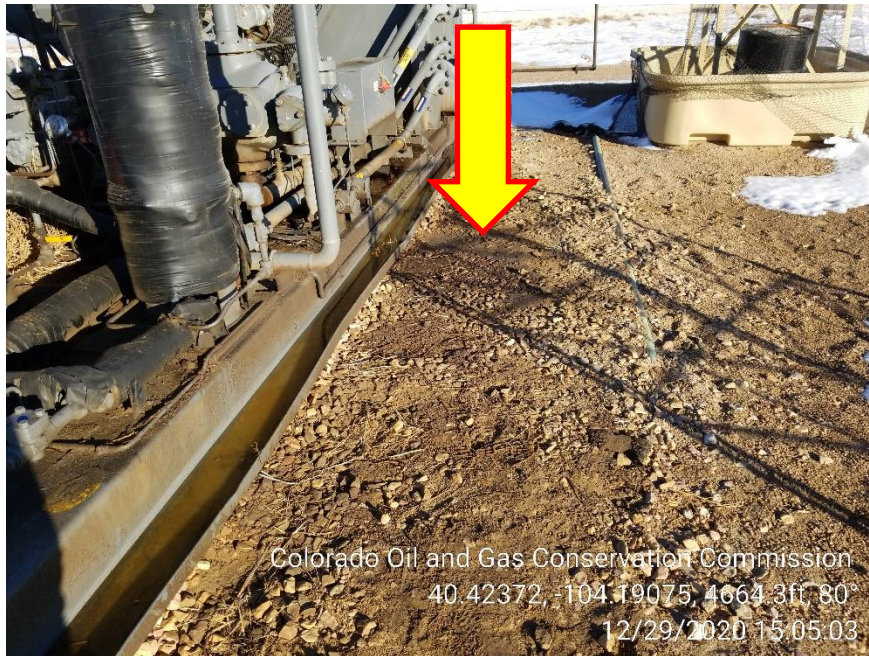
Photo 9 – Stained Soil at Compressor
