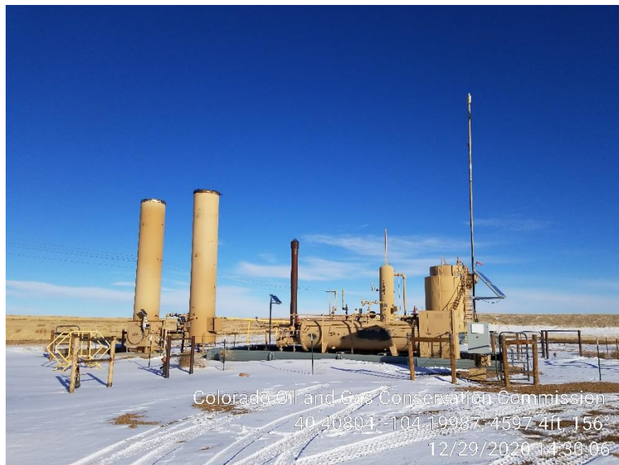
Photo 1 – Separator and ECDs
