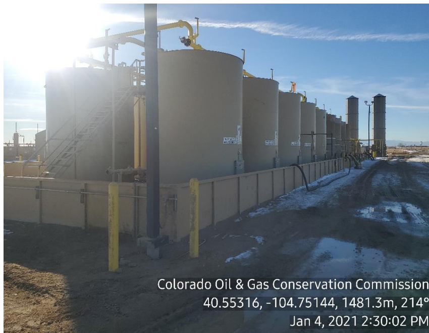
Photo 3: Tank Battery
