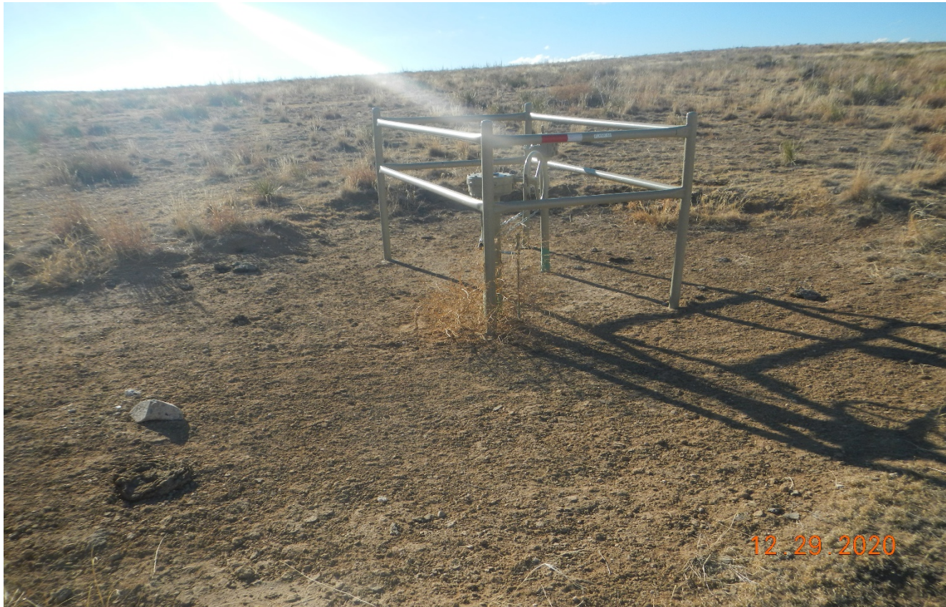
Photo 4. There is a pipe riser that remains at the west side of the location. All equipment should have been removed within 3 months of abandonment of the well.
