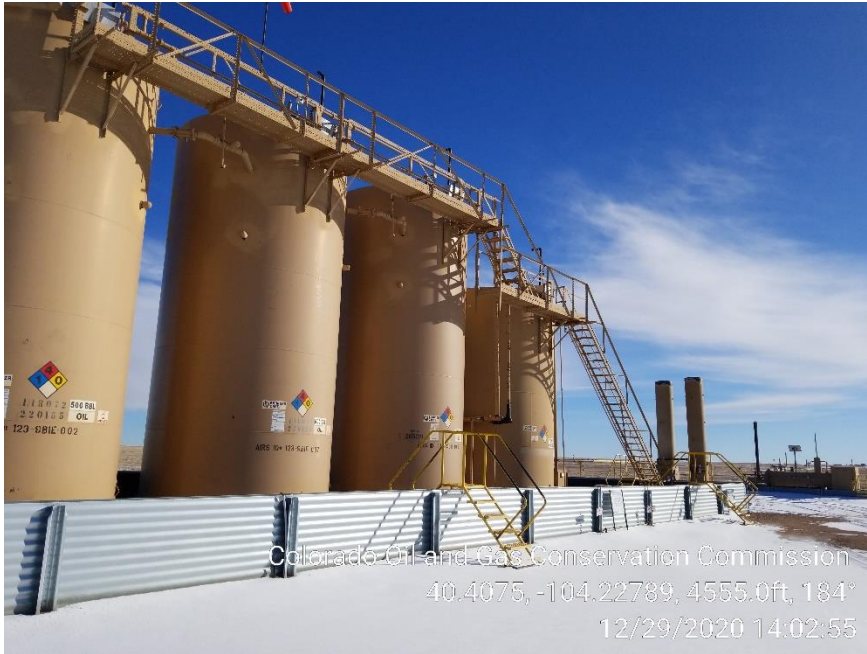
Photo 3 – Tank Battery
