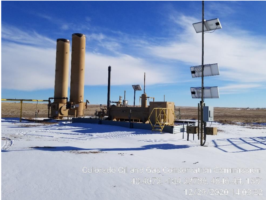
Photo 5 – Separator, ECDs
