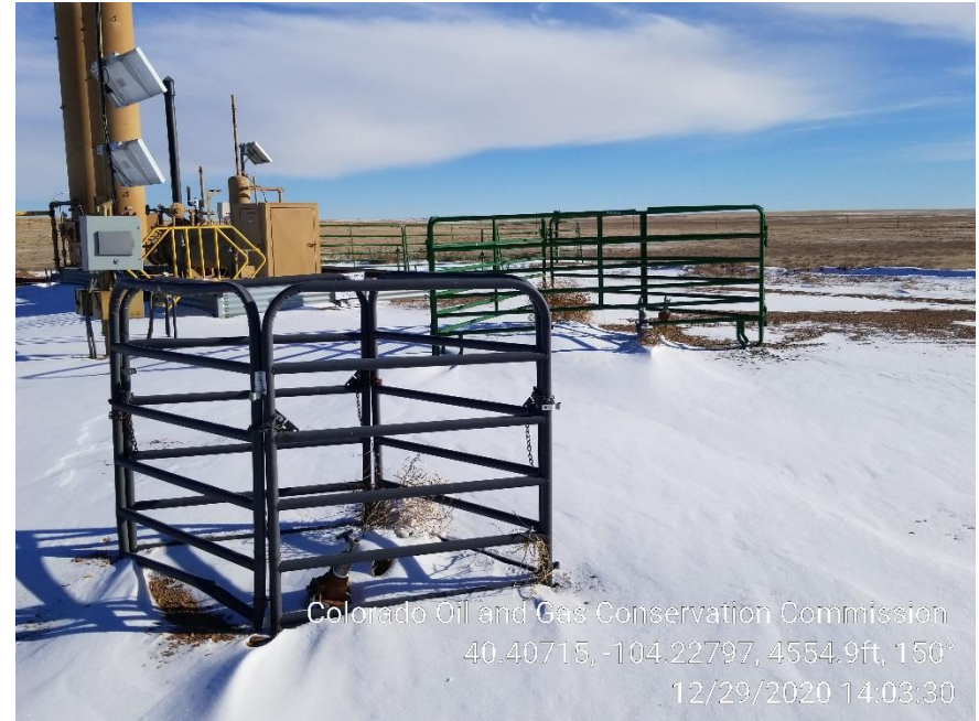
Photo 6 – Risers have been marked
