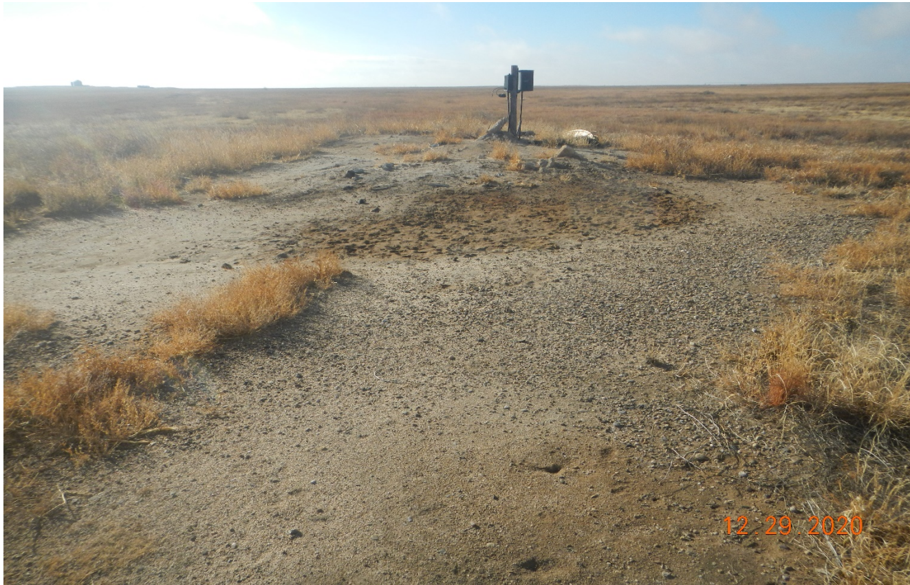
Photo 3. Facing southwest. This area has no vegetation growth and has not been regraded and leveled. Soils need to be decompacted by cross ripping to 18 inches.
