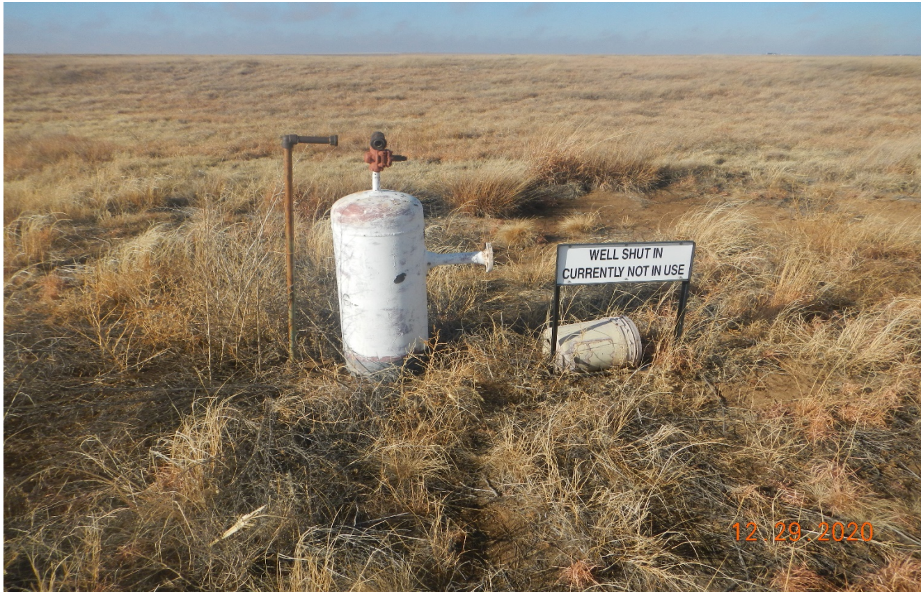
Photo 2. There is a sign, tank, and pipe riser that remains. The well was plugged and abandoned on 9/1/2017. All equipment should have been removed within 3 months of abandonment.
