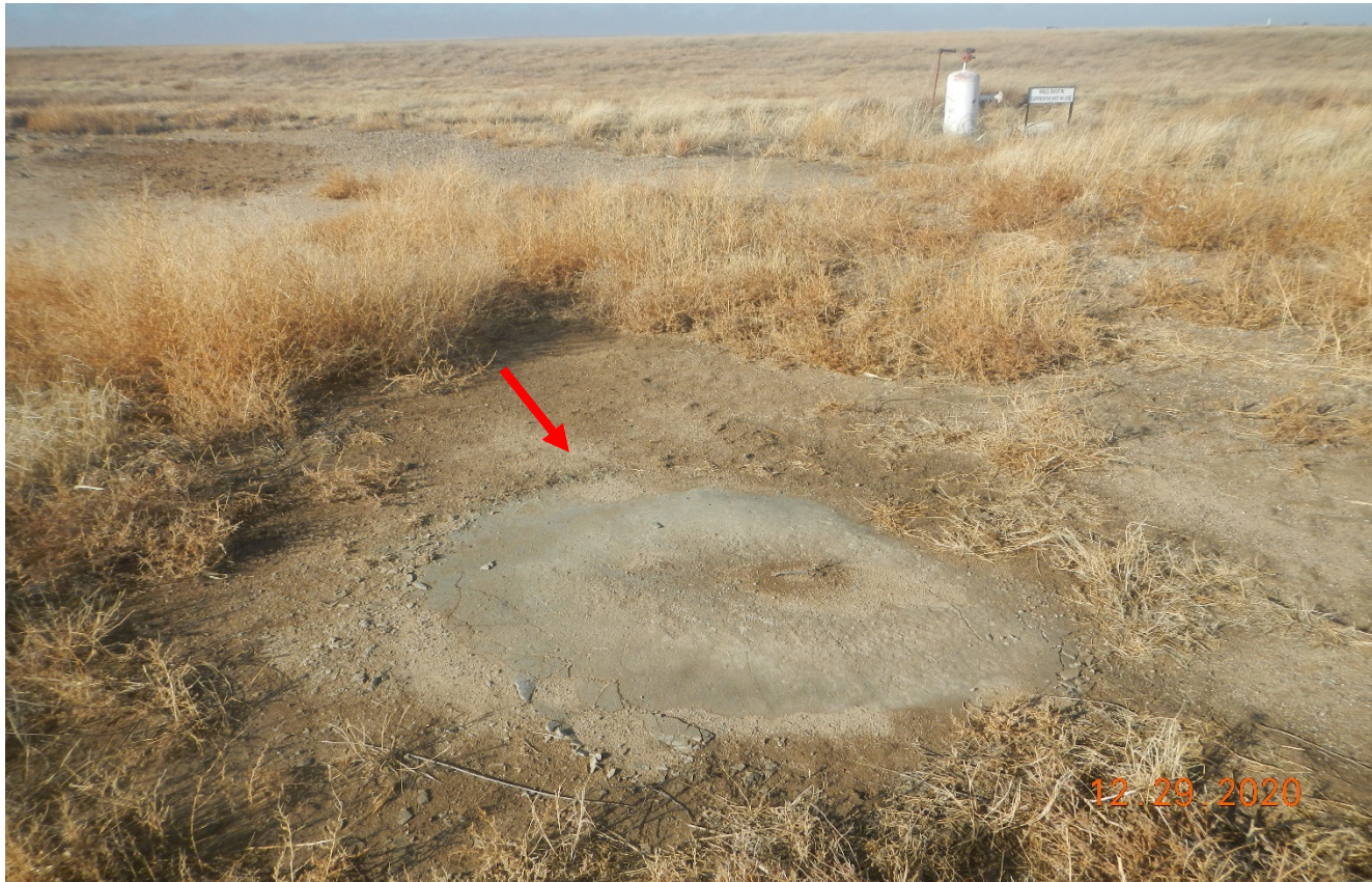
Photo 6. There is cement that remains at the east side. The cement needs to be removed.
