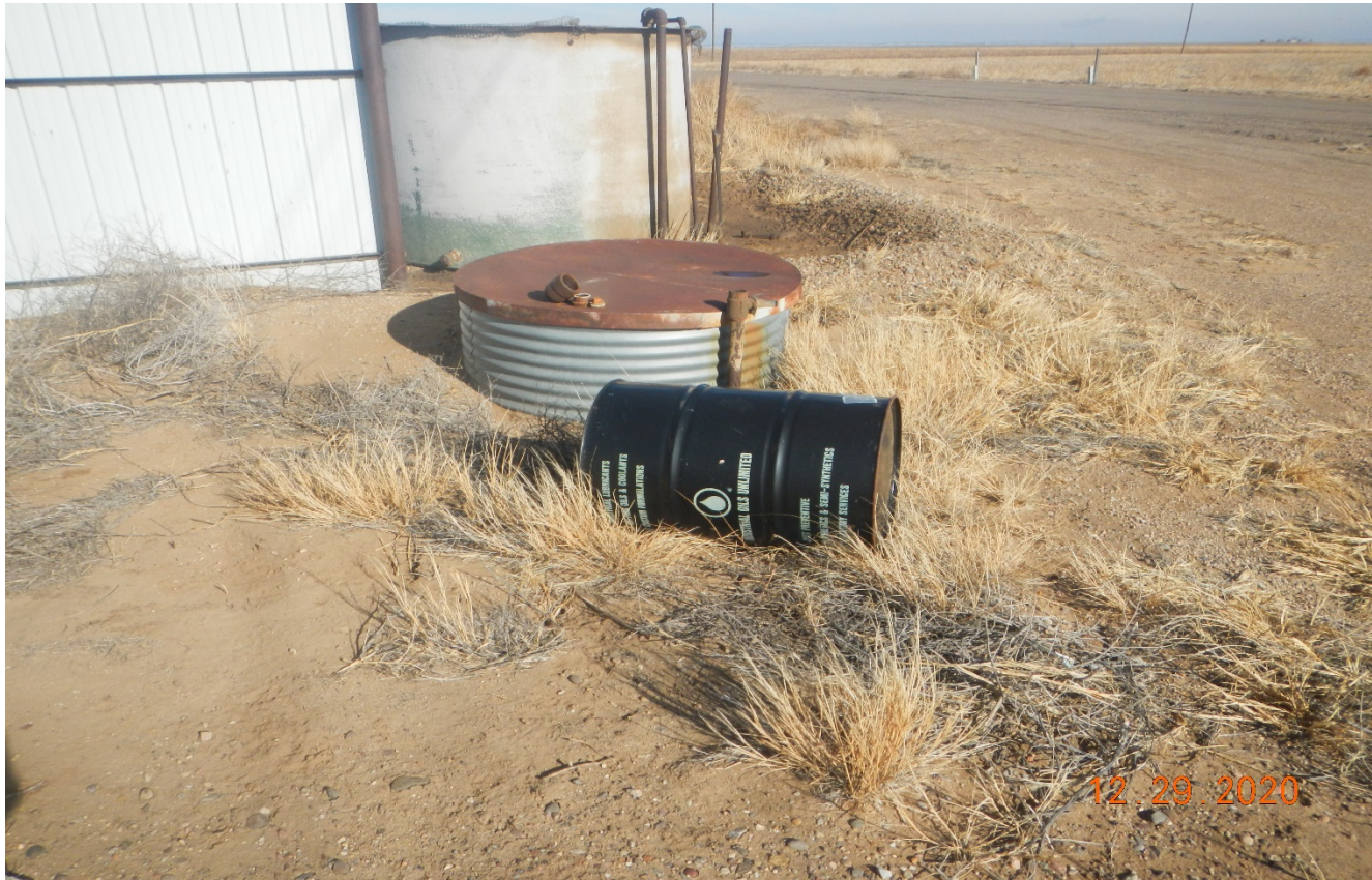
Photo 3. There is a barrel tipped over which is not sealed .
