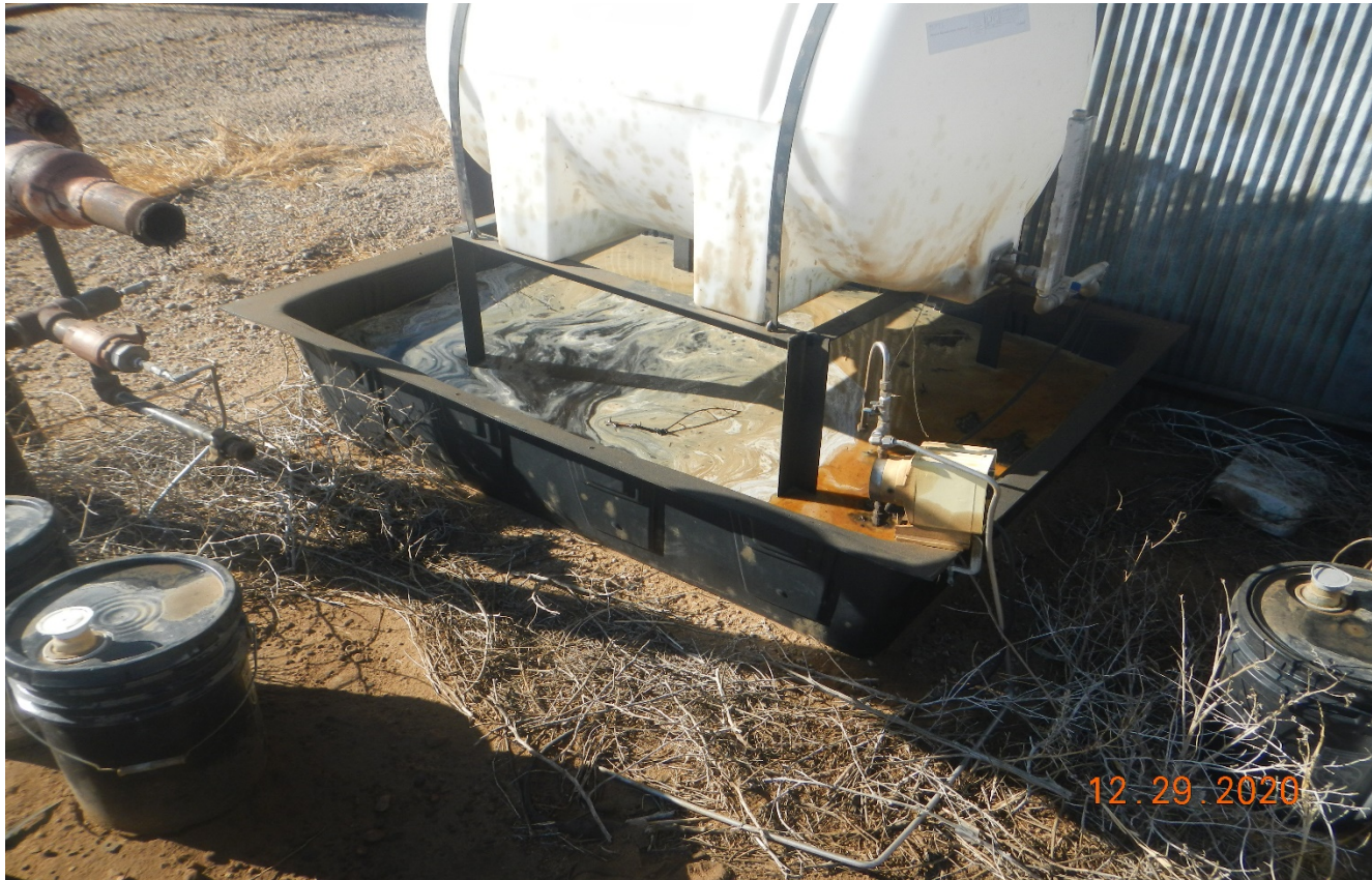
Photo 6. There is oily waste inside this containment which is near the top of the containment and appears to have spilled over.
