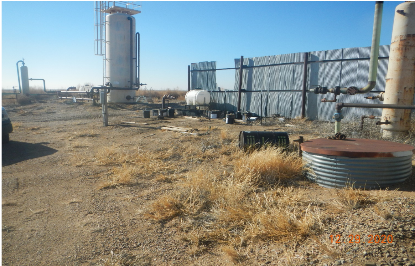
Photo 9. Facing southwest toward the location which is adjacent to County Rd. 44. The facility is not maintained and there are numerous issues observed.
