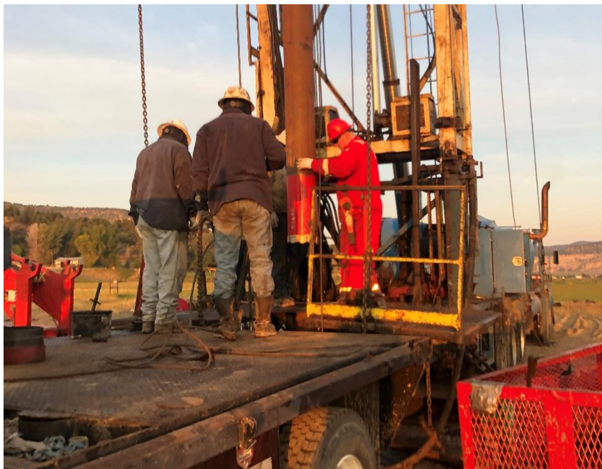
1: Running in hole with washover milling drill bit
