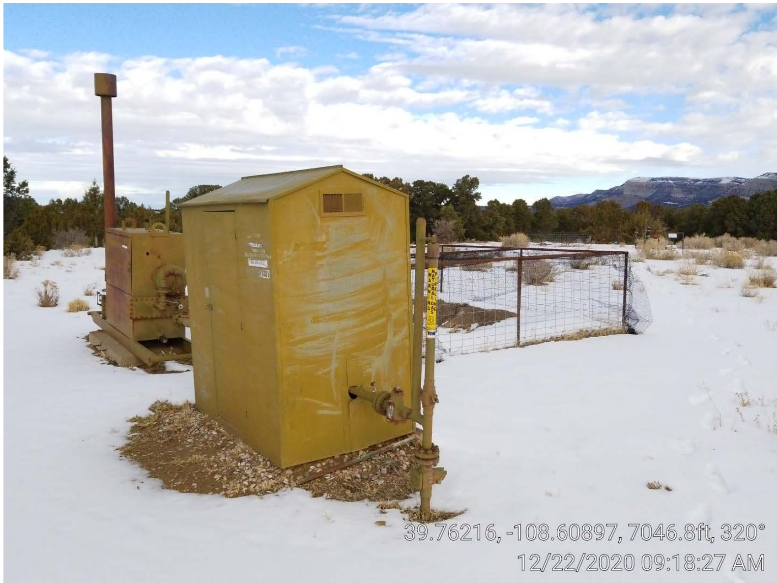
Photo 3. Meter building, separator, pit.
