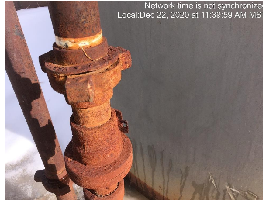
Photo #2527 Figure 200 hammer union rusted and cracked.
