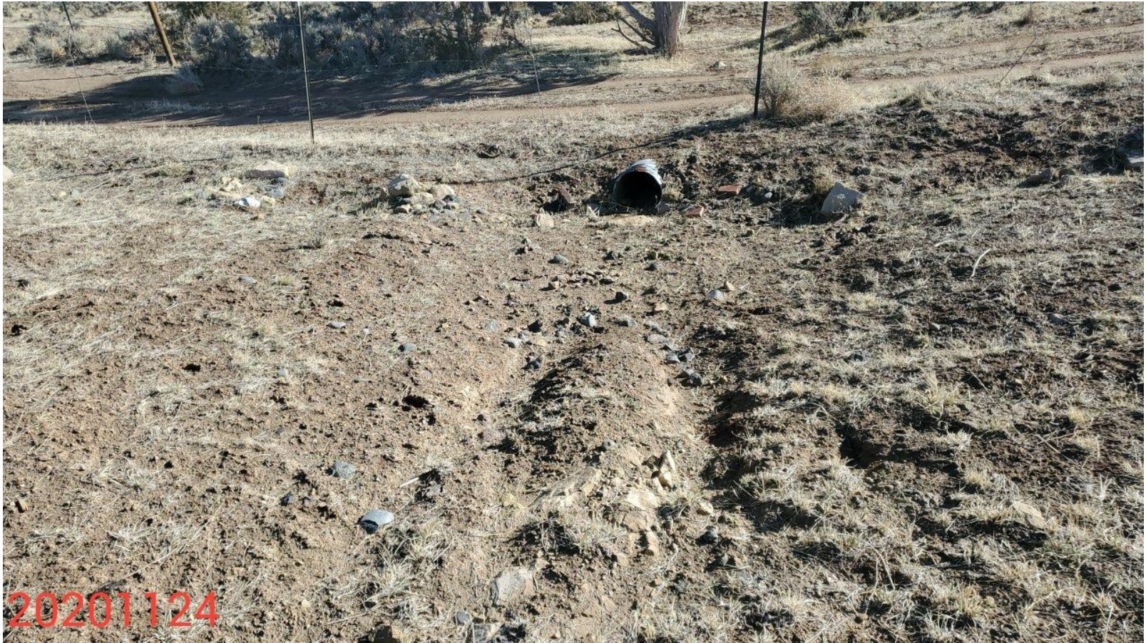
Photo 5: Photo taken from the northwest end of the Location. Photo shows culvert and drainage. Culvert has not been installed in accordance with good engineering practices and is missing proper inlet/outlet protection.
