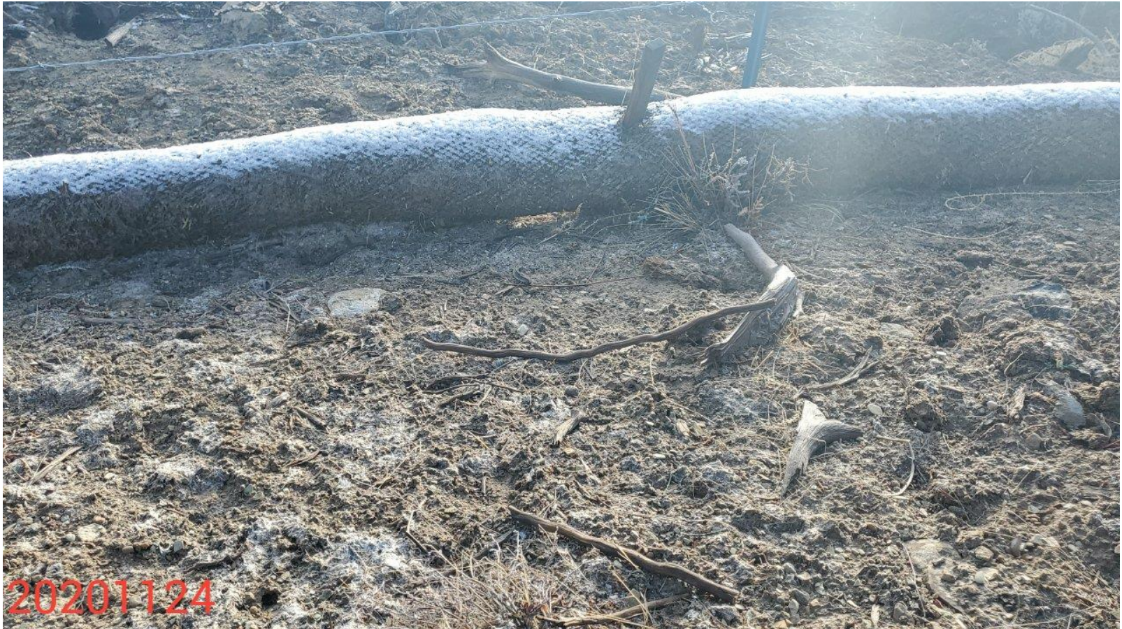
Photo 13: Continued from photo 12. Photo shows perimeter BMPs have not been installed in accordance with good engineering practices.
