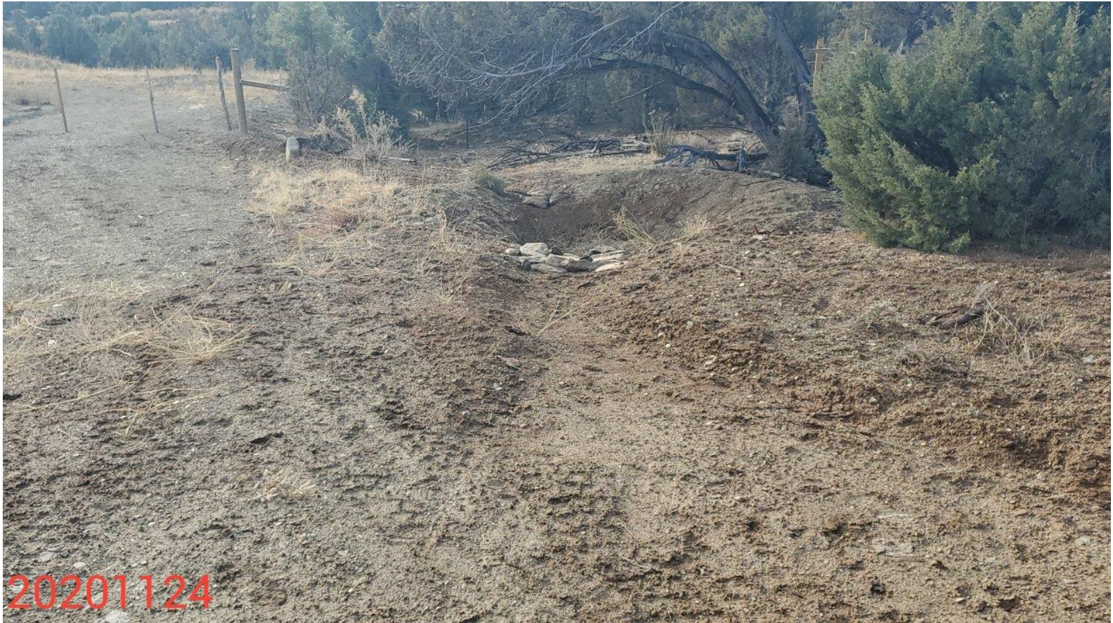
Photo 4: Photo taken from the access road, facing south. Photo shows sediment trap along access road. BMP has not been installed in accordance with good engineering practices.
