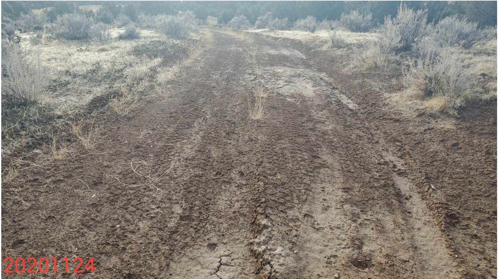
Photo 3: Continued from photo 2. Access road requires graveling. BMPs installed on/along access road need to be installed in accordance with good engineering practices pursuant to 1002.f Rules.
