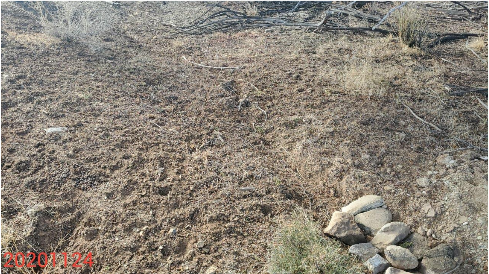
Photo 5: Continued from photo 4. Photo shows outlet at sediment trap has not been constructed in accordance with good engineering practices.
