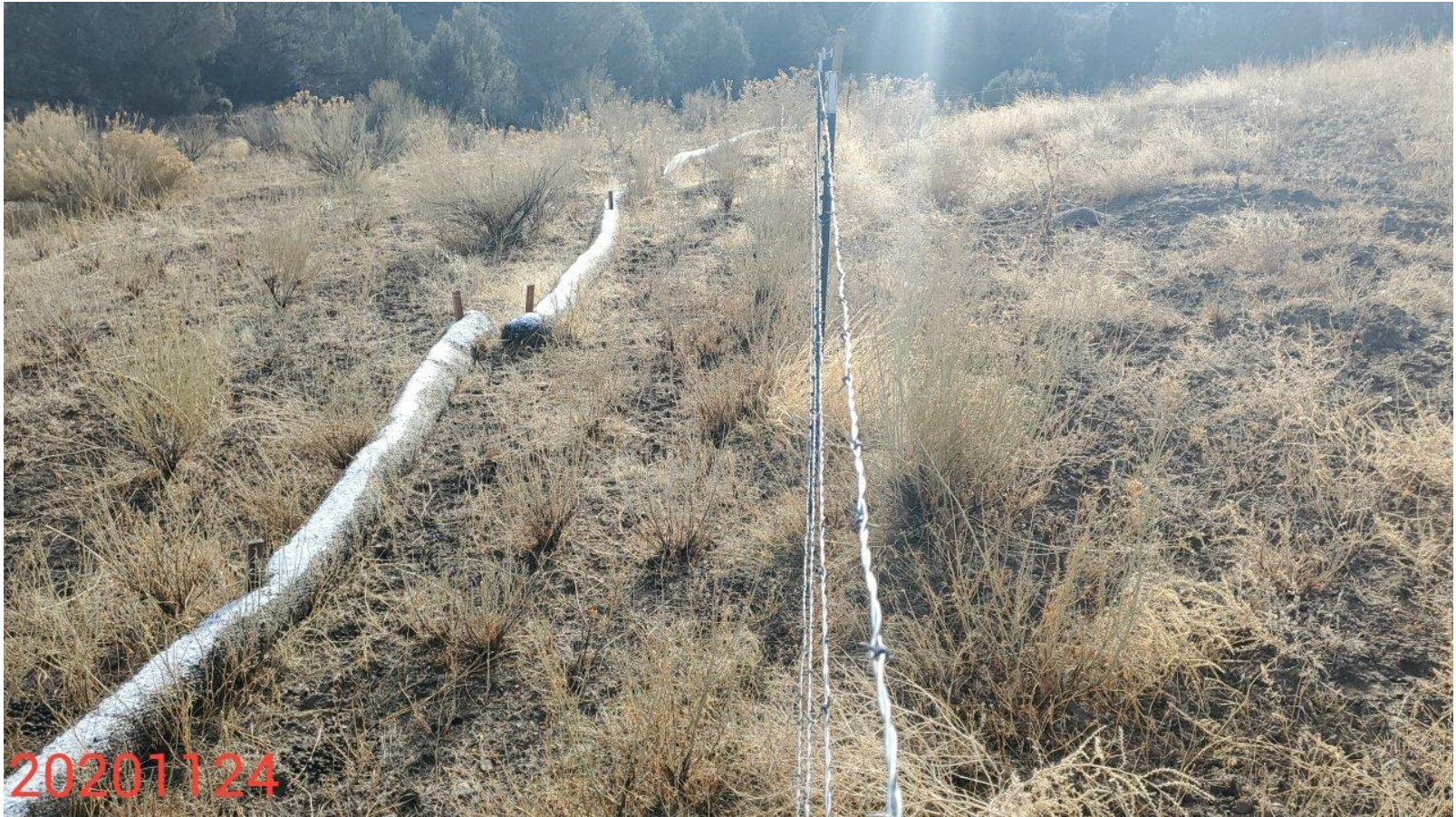
Photo 12: Photo taken from the east end of the Location, facing southeast. Photo shows example of perimeter BMPs that have not been installed in accordance with good engineering practices.
