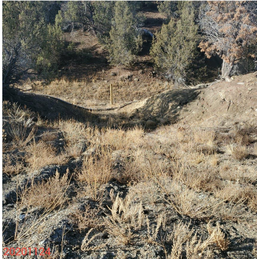
Photo 16: Continued from photo 15. Photo shows Access road at location entrance was constructed in a manner that dammed a drainage on the west end of the Location; BMPs missing or insufficient to allow water movement within the drainage. Access road requires graveling. Photo also example of BMPs missing, or insufficient to stabilize slopes of the Location.
