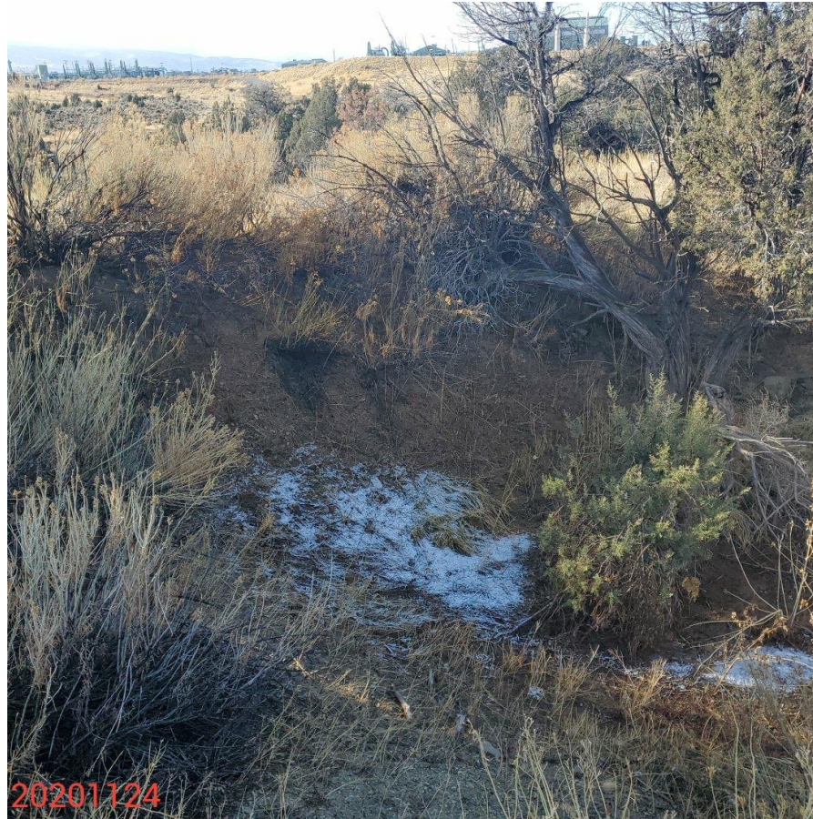
Photo 15: Photo taken from the northwest end of the Location, facing west. Photo shows Access road at location entrance was constructed in a manner that dammed a drainage on the west end of the Location; BMPs missing or insufficient to allow water movement within the drainage. Access road requires graveling
