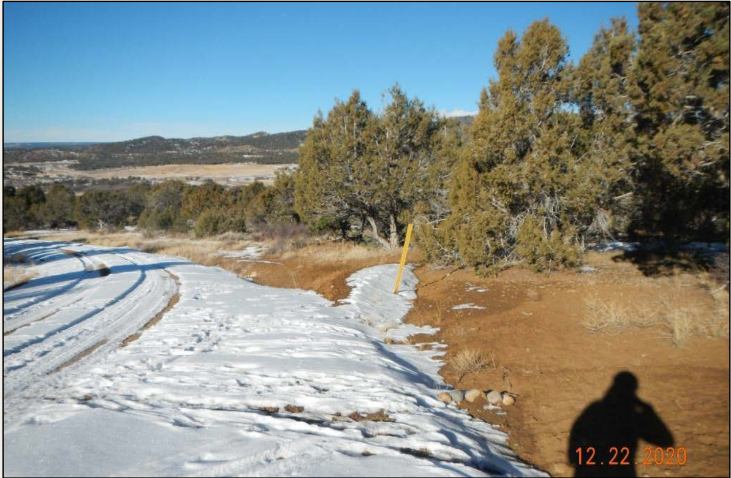
Photo 4. View of cobble along roadside drainage full of sediment. BMP is not adequate here.
