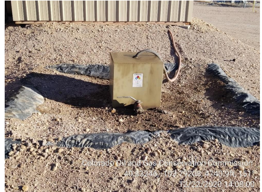
Photo 6 – Stained Soil at Condensate Tank
