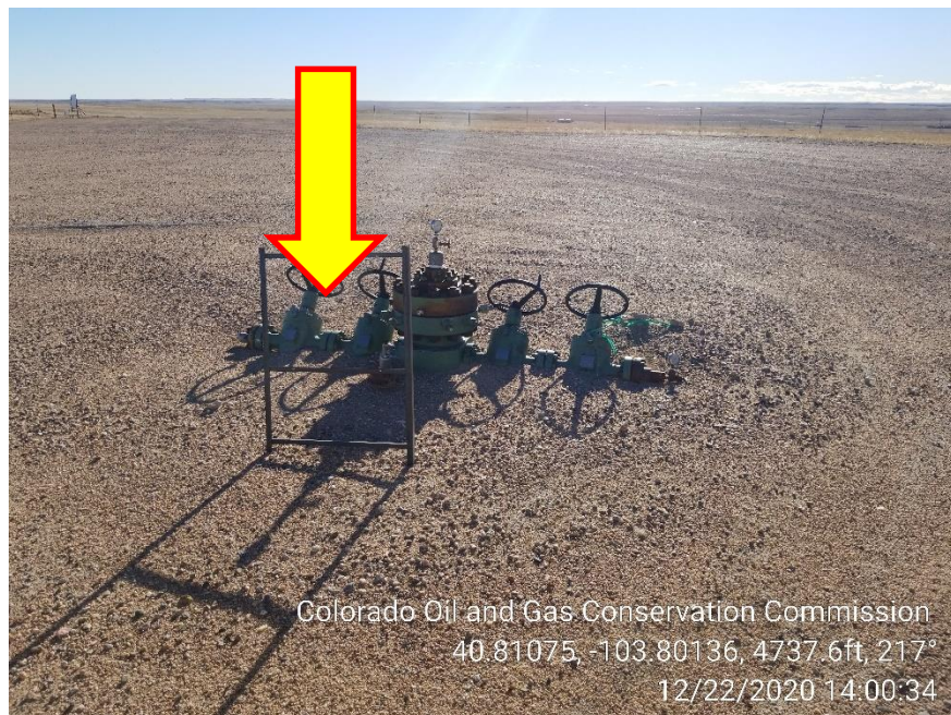
Photo 3 – 30E-1934 missing Wellhead Sign
