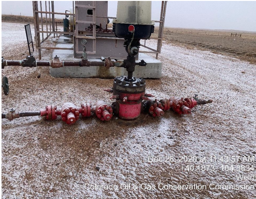
Photo #7 Surface Casing has no Bradenhead provisions (Not Plumbed to Surface)
