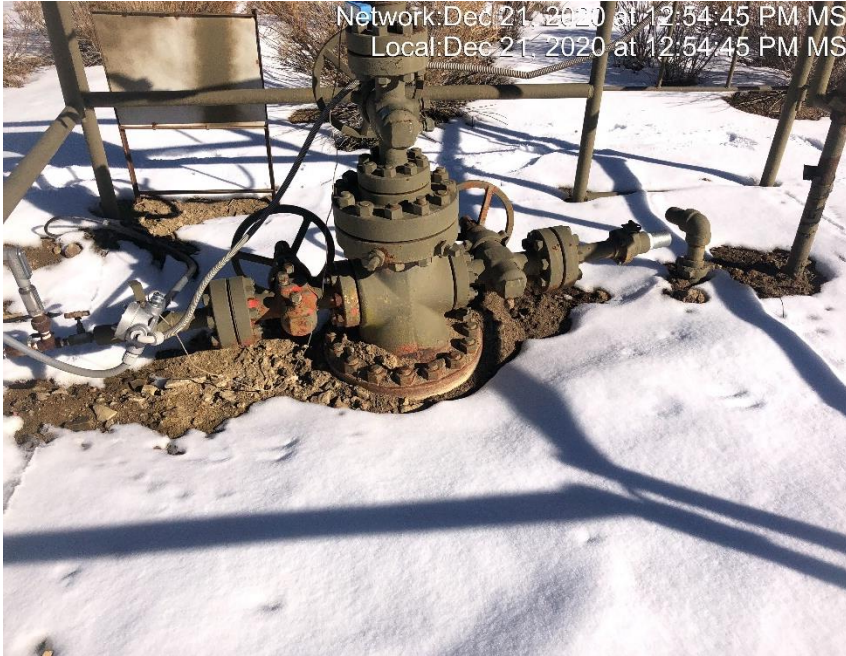
Photo #2510 Braden head valves are not accessible.
