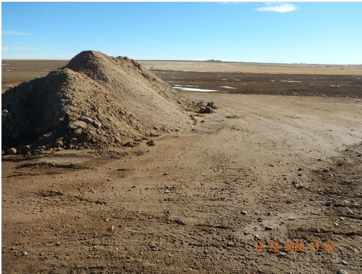
Photo 1. Photo taken from the southern tank battery location, facing East. Photo illustrates Operator has failed to removed all gravel and perform final reclamation activities.
