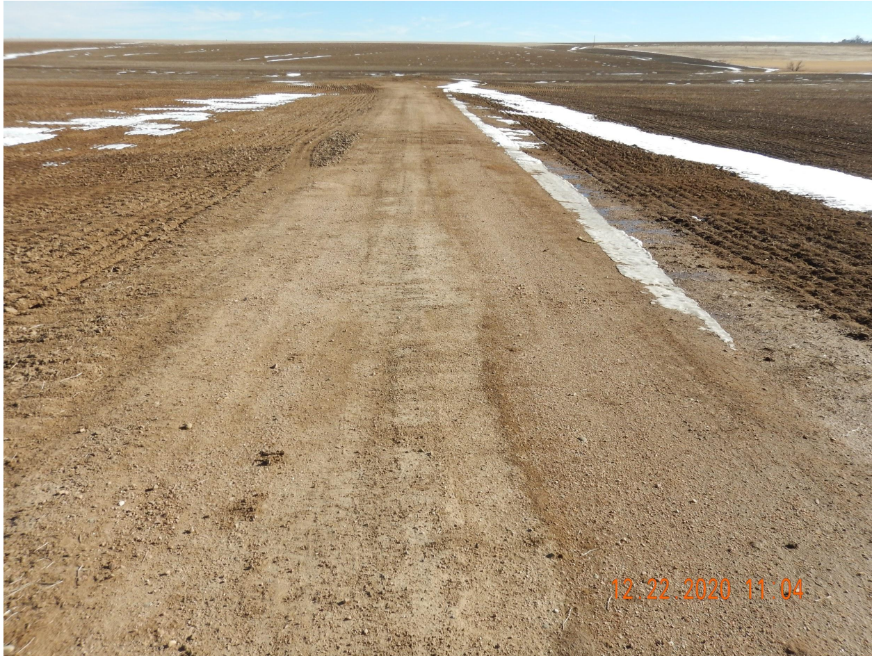
Photo 3. Photo taken from the well location access road, facing East. Operator has failed to properly contour and perform final reclamation activities.
