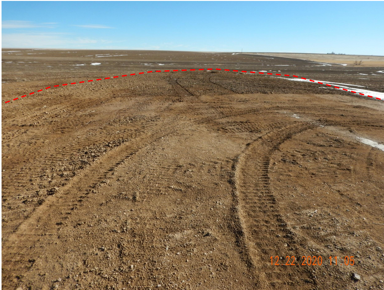
Photo 4. Photo taken from the well location, facing East. Operator has failed to properly contour and perform final reclamation activities.
