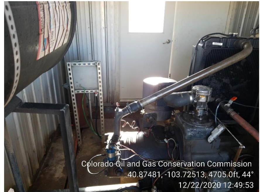
Photo 8 – Stained Soil at Gas Engine
