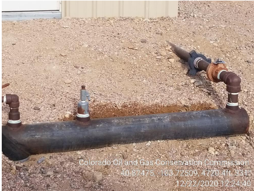
Photo 7 – Stained Soil at Supply Pot
