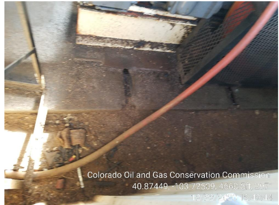
Photo 8 – Stained Soil at Gas Engine
