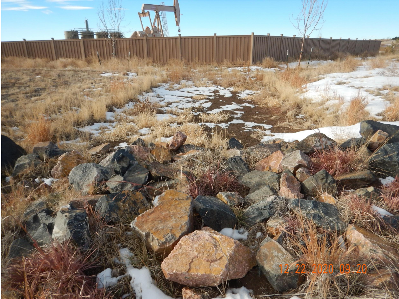
Photo 3. Photo taken from the northeastern location, facing Southwest. Photo illustrates a sediment trap which appears to be in proper functioning condition at the time of this inspection.
