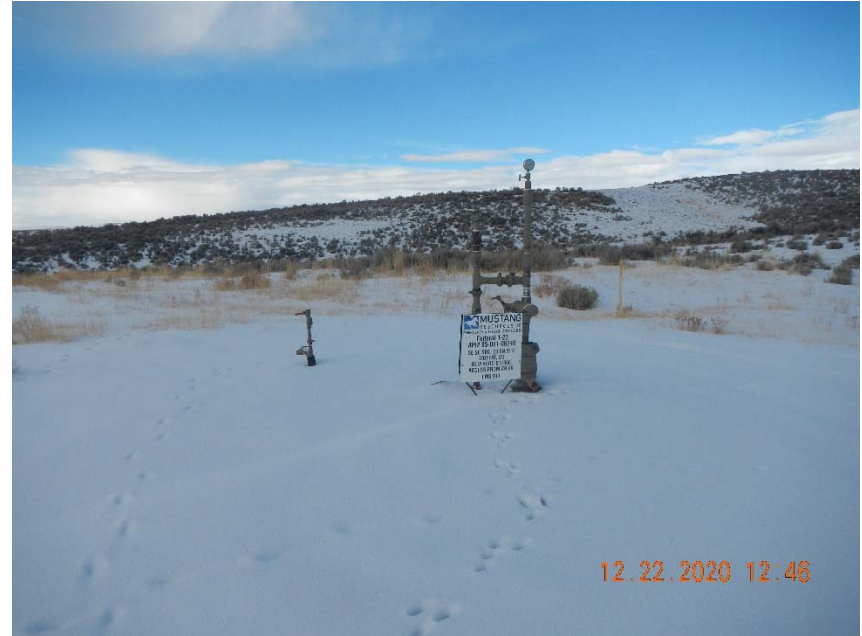
Photo 2. Previous operator and contact information on location signs. No bradenhead access apparent.
