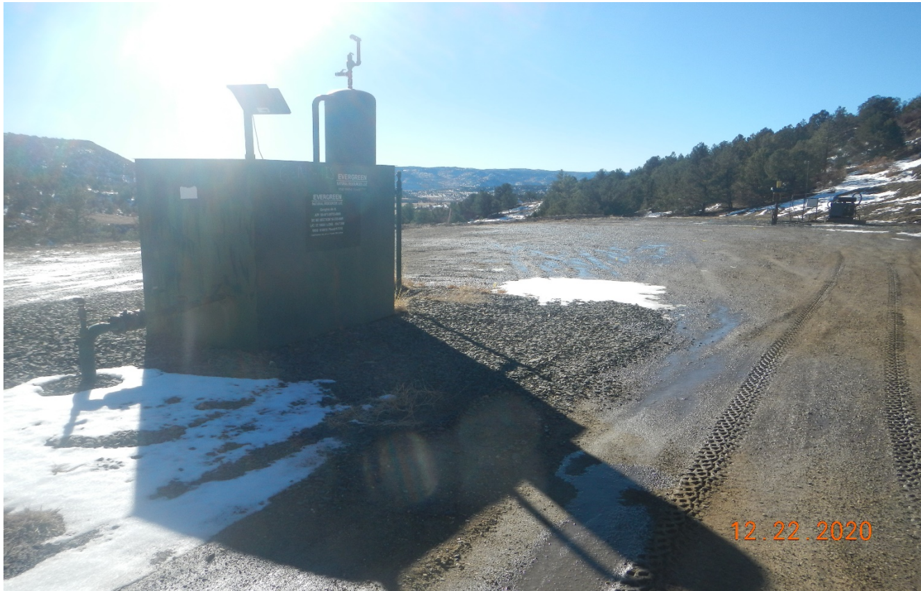
Photo 1. Facing southeast toward the location.
