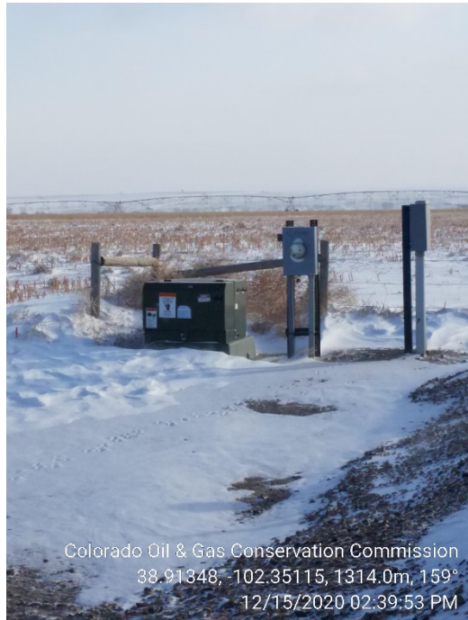
5. Transformer, Elec panel, elec meter
