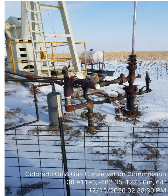
4. Wellhead scrubber, line heater manifold
