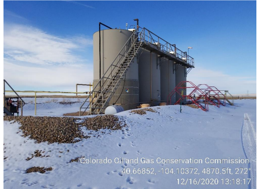
Photo 6 – Tank Battery
