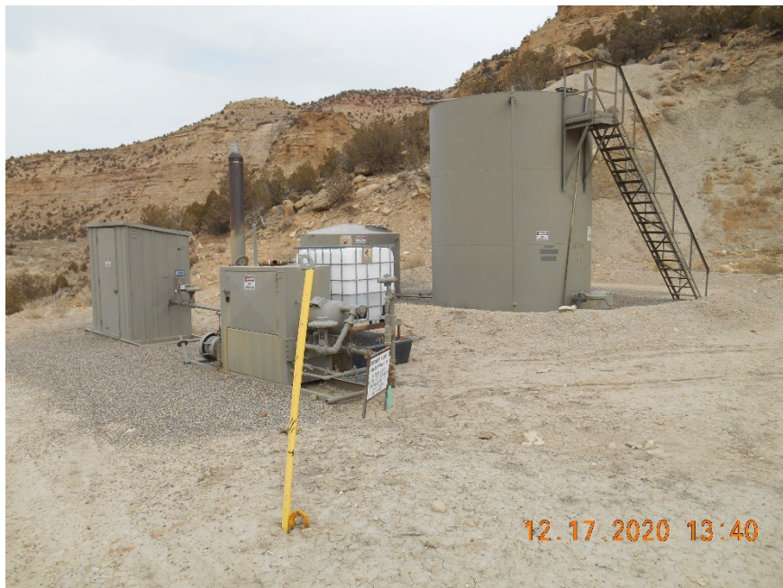
Separator, Meter housing and Tank Battery
